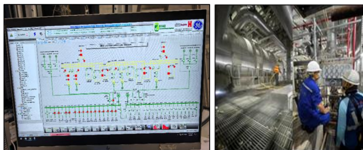
Fig. 15 - Connecting to Grid (Left) & Commissioning of Power Island (Right)
