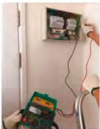
Electricity and Safety by CHEUNG Hon Lun
