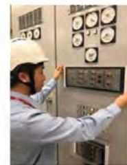
Preparation for Secondary Injection Test on Auto-Syn relay
