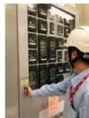
Preparation for Protection System Isolation
