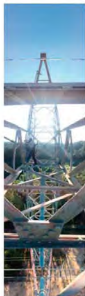
Overhead Line Training on Transmission Line Tower by LI Hoi Ching
