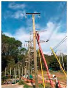
Overhead Line Training by LI Hoi Ching
