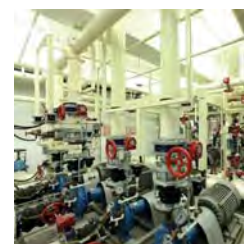
Fire Services & PD
