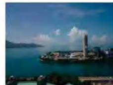
Generation Substation by CHAN Chun Pui, Brian
