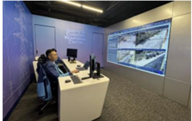
Fig. 3 - CLP Power’s Grid Visualisation (Grid-V) Control Centre for monitoring Critical Assets
