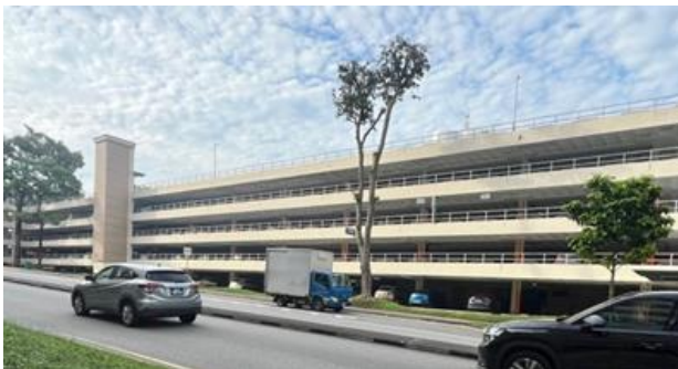
Fig. 5 - Singapore Public Housing Carpark CLRG (HDB Block 312 Multi-Storey Carpark) with PSN
