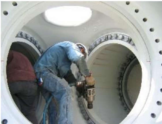
Fig. 6 Adjustment of the pitch angle to the required value by loosening and re-tightening the bolt.
