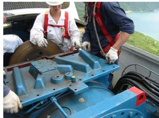
Fig. 5 Routine Maintenance of Wind Turbine
