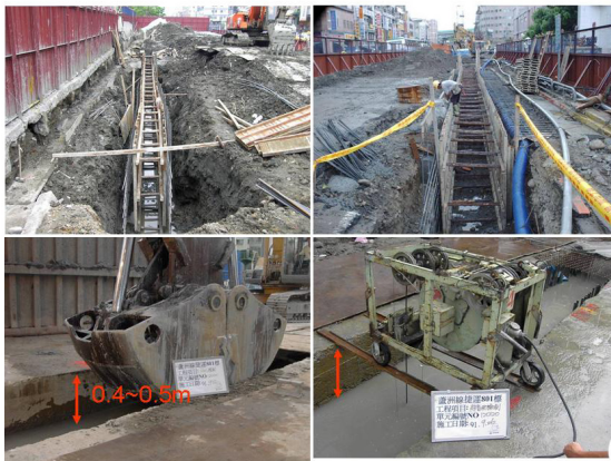
Figure 3-6: Slurry controlled at 0.4m below guide wall surface for O46 station.
