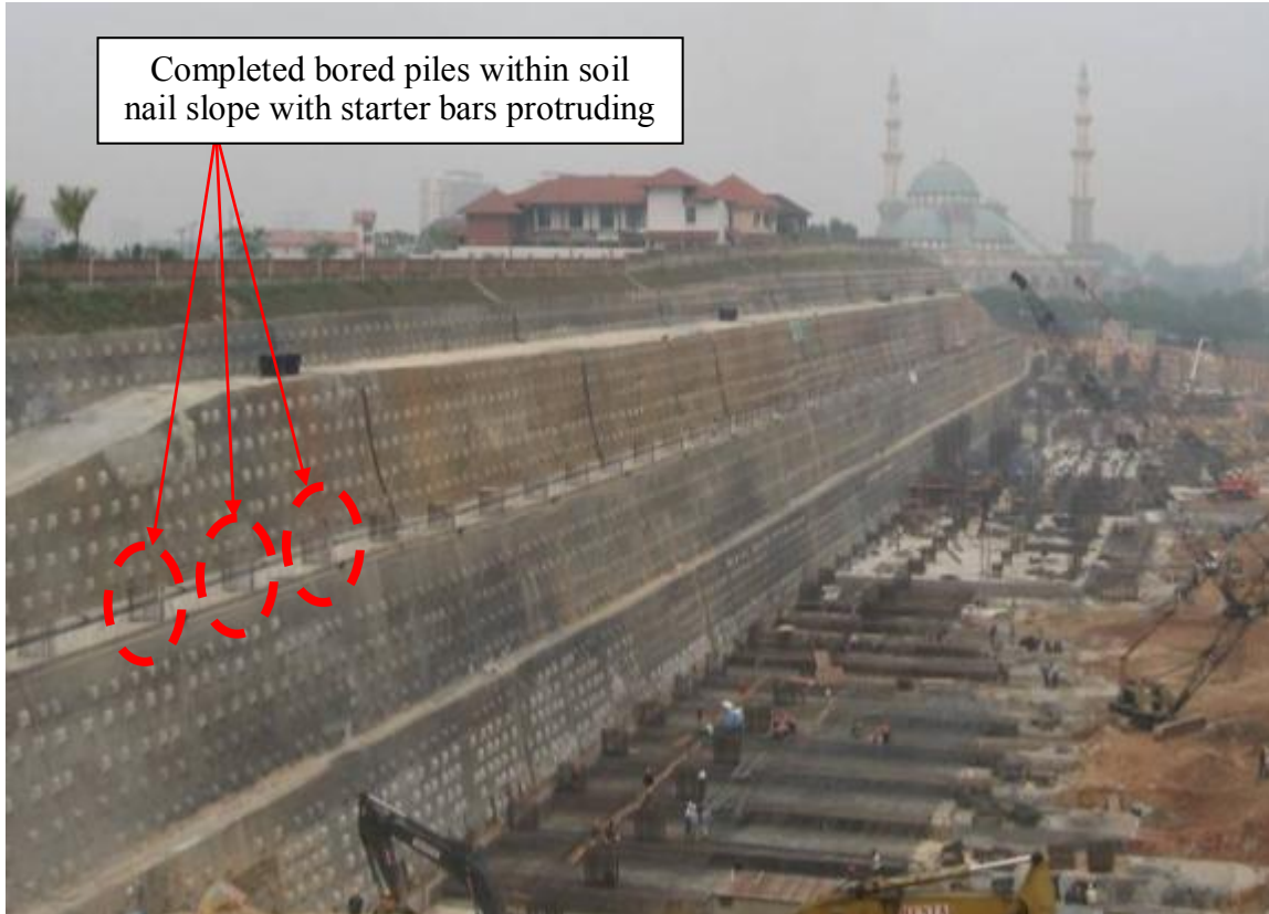
Figure 9: Picture taken after completion of soil nailing works and basement construction on-going.
