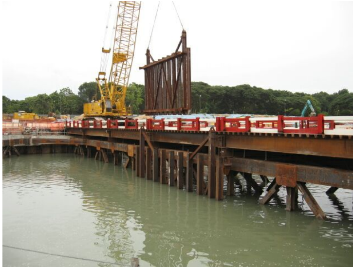
Plate 2: Fender panels for the protection of temporary earthwork supports
