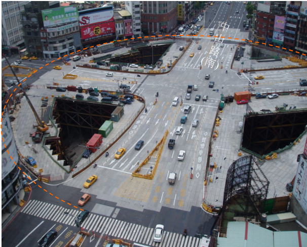
Figure 5.1: Status of the internal circular excavation
