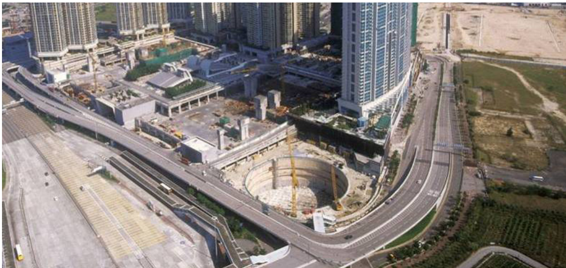
Plate 4: Overview of the excavation for the International Commerce Centre
