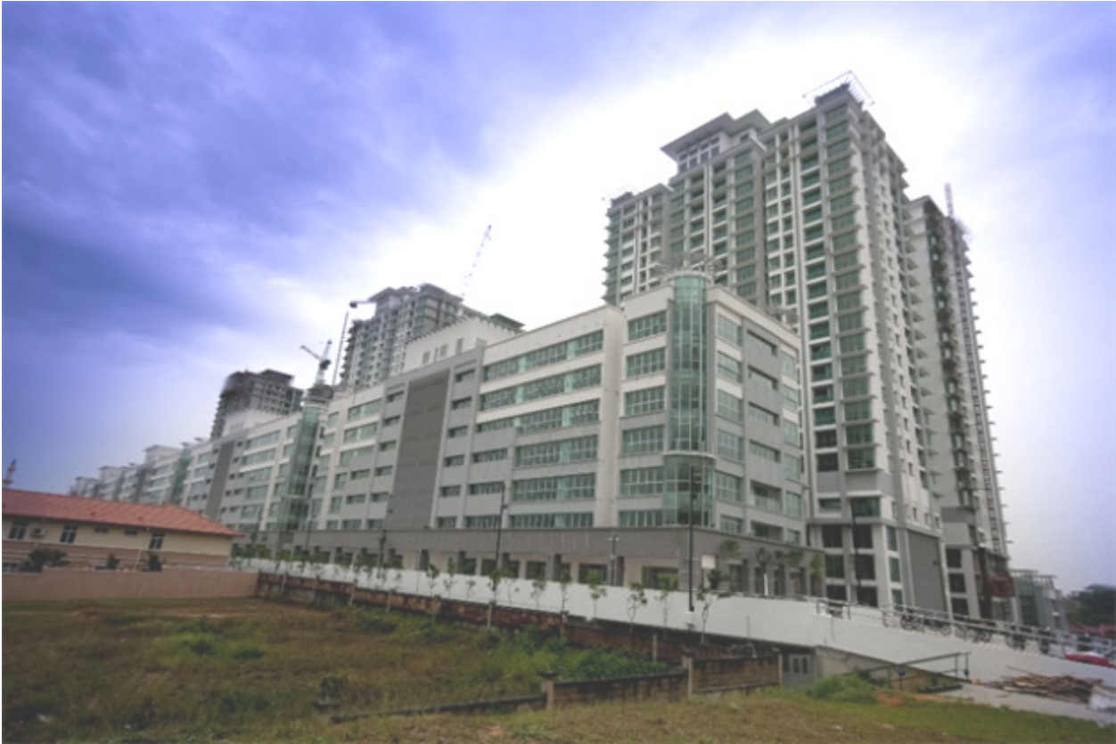
Figure 3: Completed basement and superstructure works.
