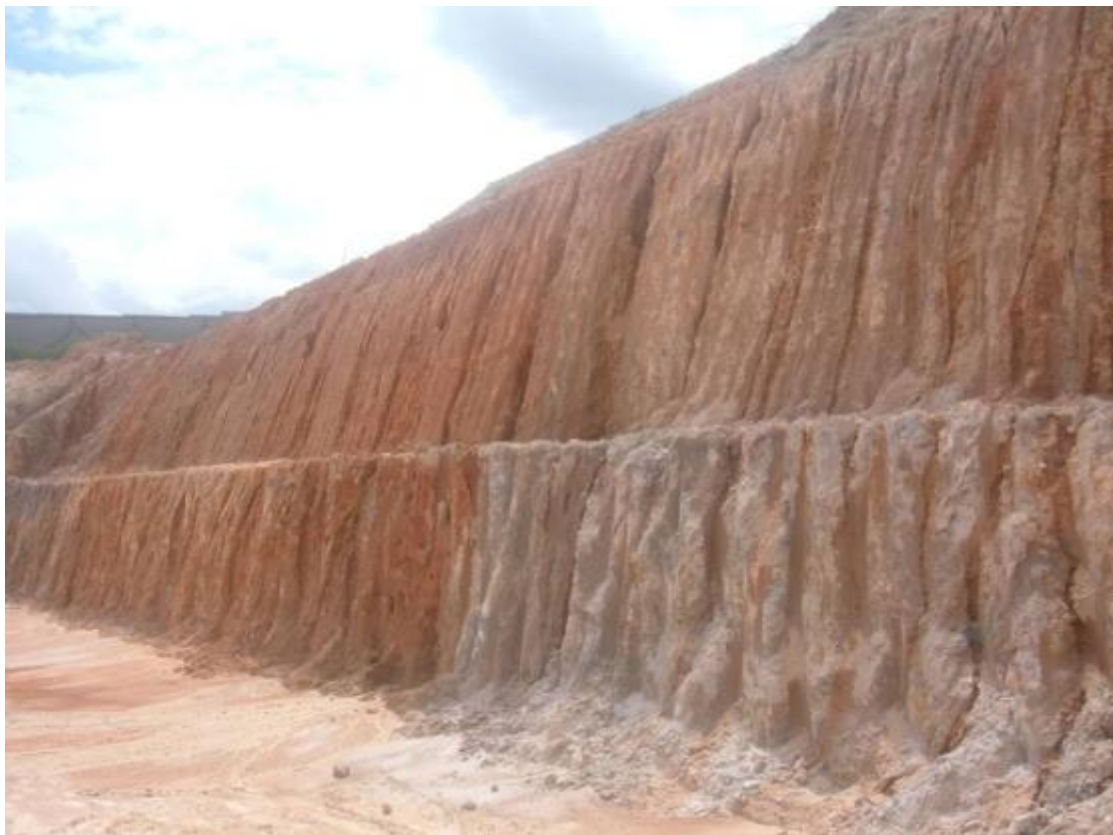
Figure 5: Typical weathered metasedimentary materials exposed during soil nail construction (Grade V/VI).
