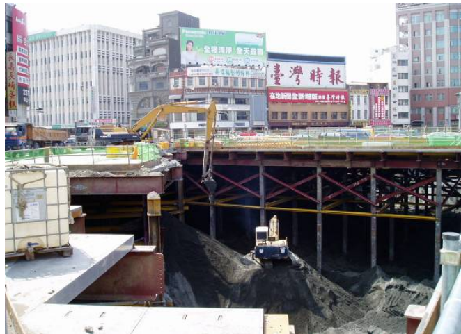
Figure 5.2: Internal excavation (GL-10m)
