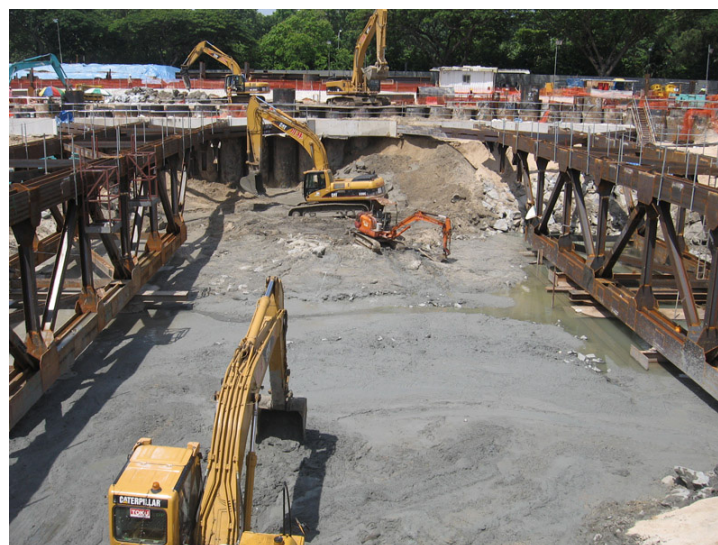
Plate 1: Maximising working space and prefabrication
