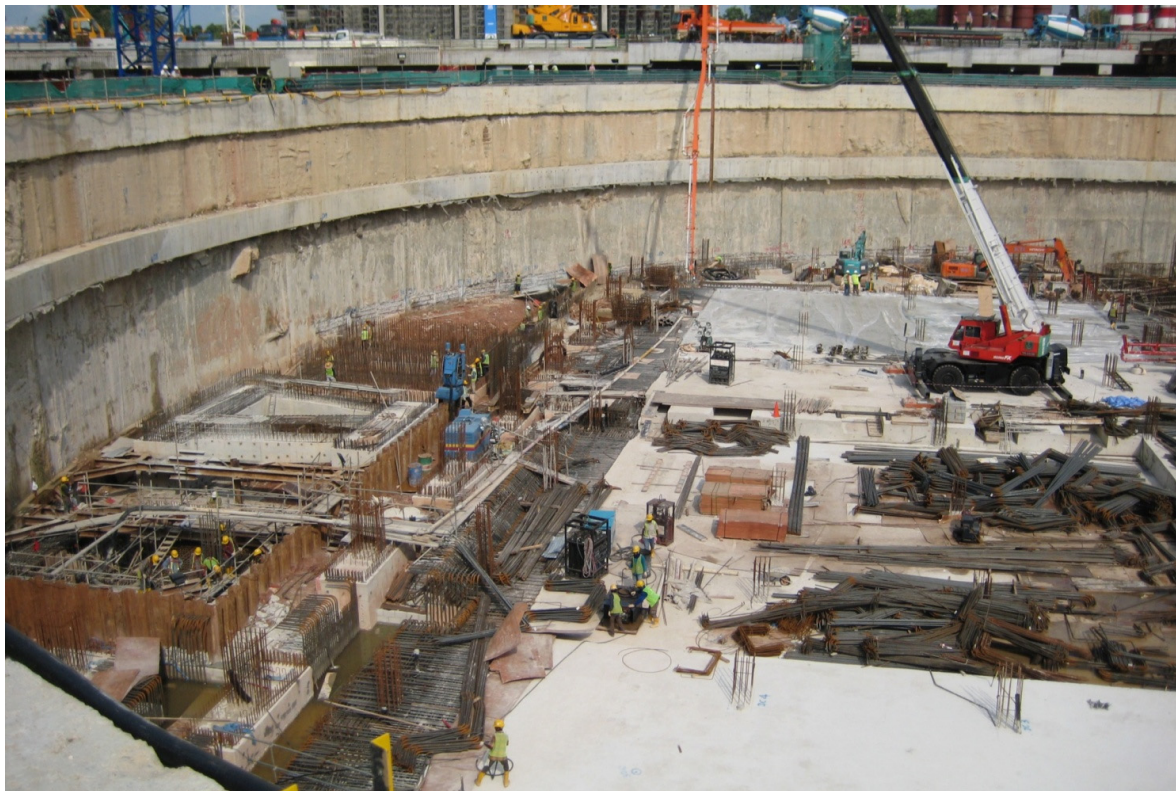
Plate 7: View within the excavation of the northern 120m diameter circular excavation
