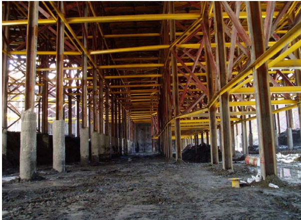
Figure 5.3: Internal excavation (GL-23.5m)
