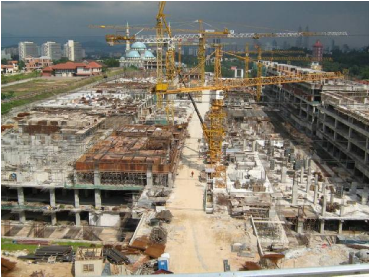
Figure 11: Picture taken after completion of basement construction.
