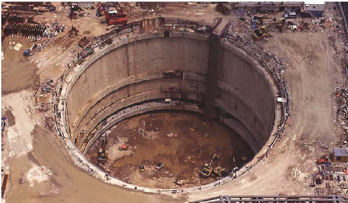
Plate 3: View of the excavation for the International Finance Centre 2
