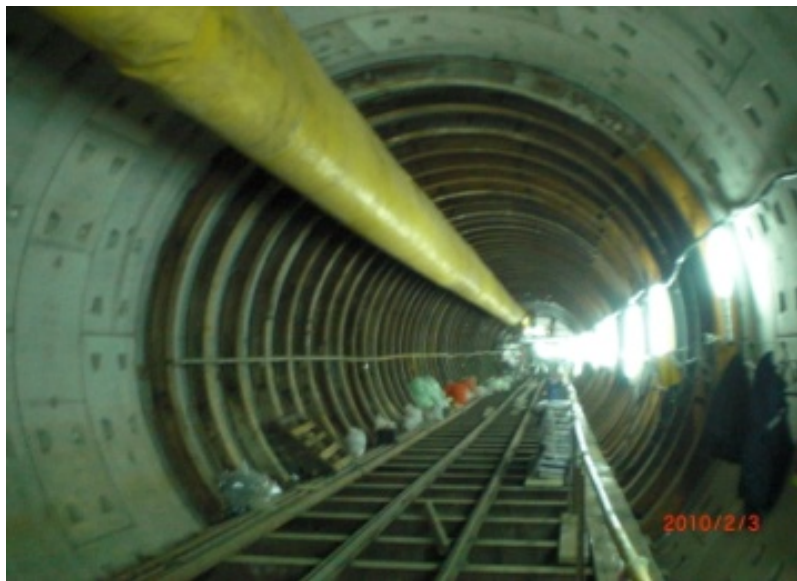
Plate 1: Tunnel propped with steel frames
