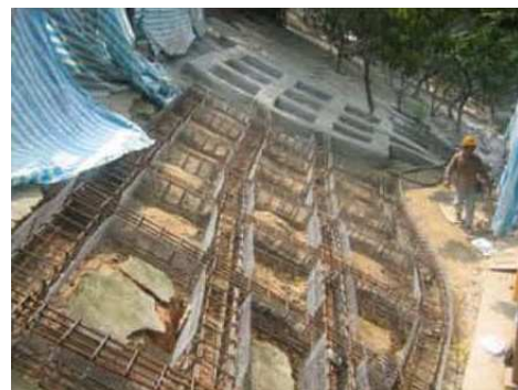
Plate 9: Pre-fabricated formwork system for concrete grillage construction
