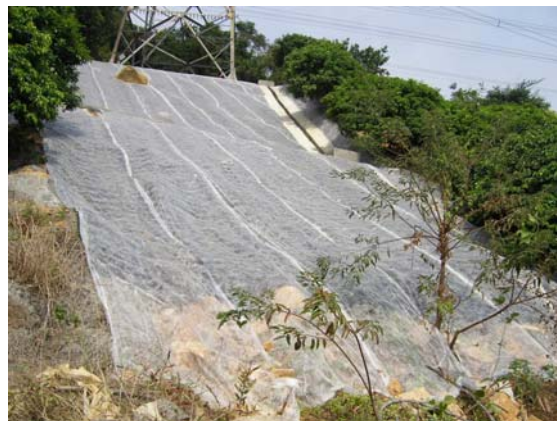
Plate 5: General View of Upgraded Slope
