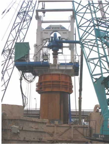
Plate 1: RCD mounted on casing top
