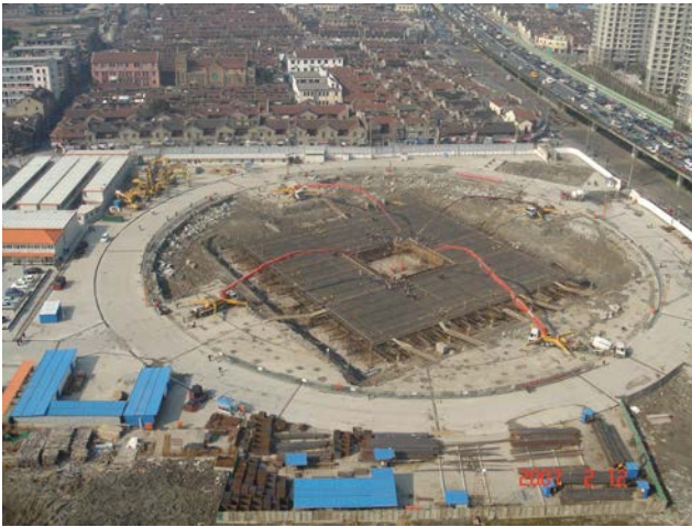
Figure 17: Pouring concrete of the central part of the roof slab
