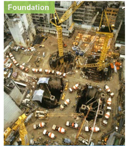
Innovation: Complex Foundation System and Associated Trial Pile Programme
