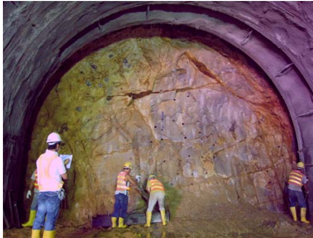
Plate 2 : Steel support frames and shotcrete lagging at portal access tunnel
