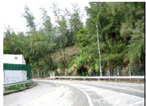
Plate 1: Felling of Trees at Castle Peak Tunnel
