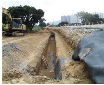
Plate 4: Trench in fine soil
