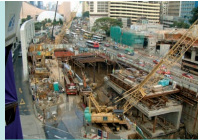
Tsim Sha Tsui KCRC Extension Hong Kong
