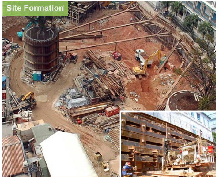
Innovation: Precise Installation of Tie-back System by Horizontal Directional Drilling
