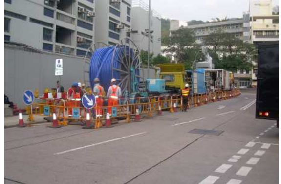
Watermains Trenchless Rehabilitation Works
