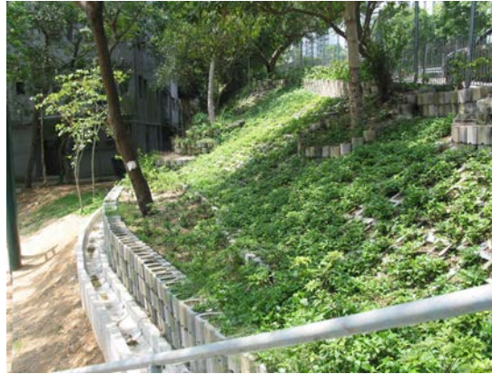
Plate 2: Slope with loose fill replaced by rubber soil
