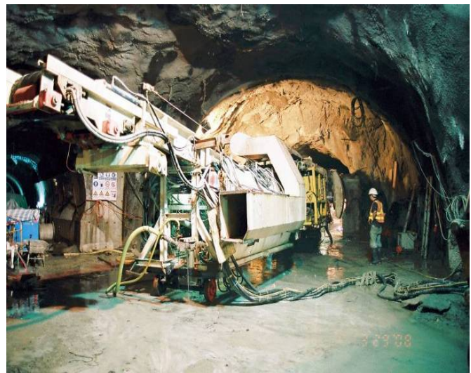
TBM Retracted to the Portal Chamber from Low Tunnel
