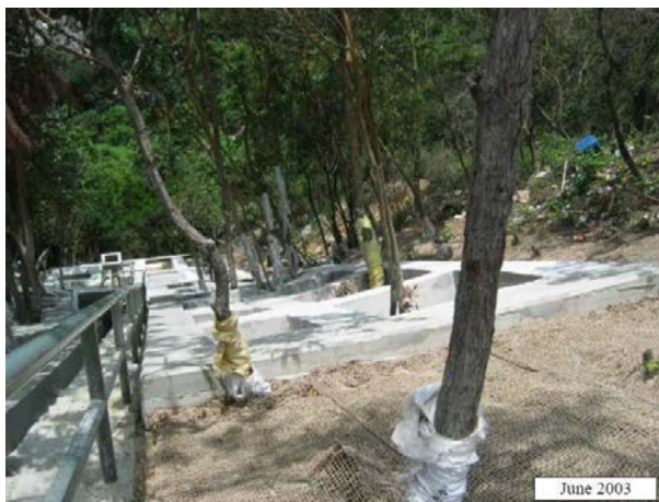
Plate 1: Completed LPM project taken in 2003 & 2007 using the concrete grillage/soil nail system
