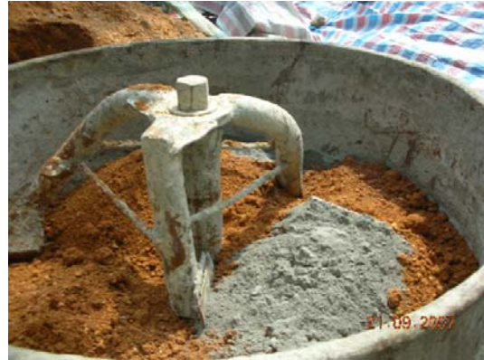
Plate 4: Photo of Electric Mixer Used on Site
