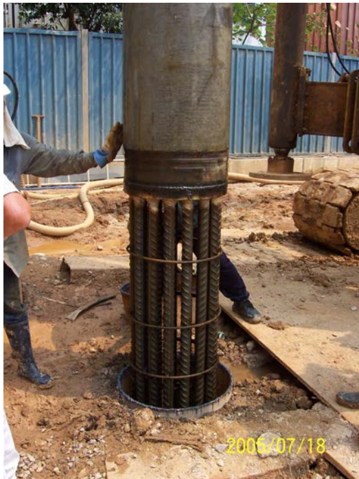
(a) (b) Figure 2: (a) Reinforcement cage and Spun pile being placed in pile bore (b) A bundle of reinforcing bars installed inside a Spun pile
