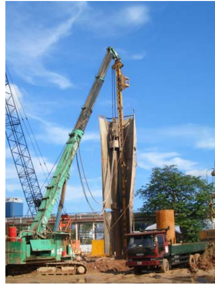
Plate 2: Pre-bored H-pile construction
