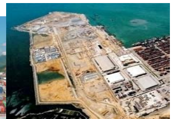
Innovation: Mud Pool Treatment by Dynamic Replacement Method
