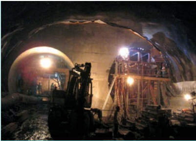
Queensway Subway Hong Kong
