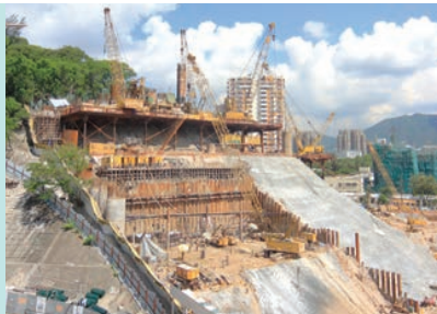
Sheung Shing Street Redevelopment Hong Kong
