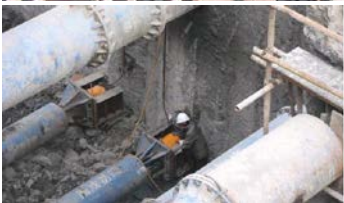
Innovation: Automatic Strut Load Compensation and Displacement Control System
