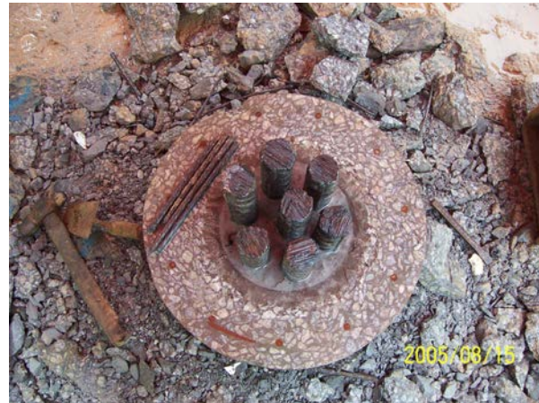
(a) (b) Figure 2: (a) Reinforcement cage and Spun pile being placed in pile bore (b) A bundle of reinforcing bars installed inside a Spun pile
