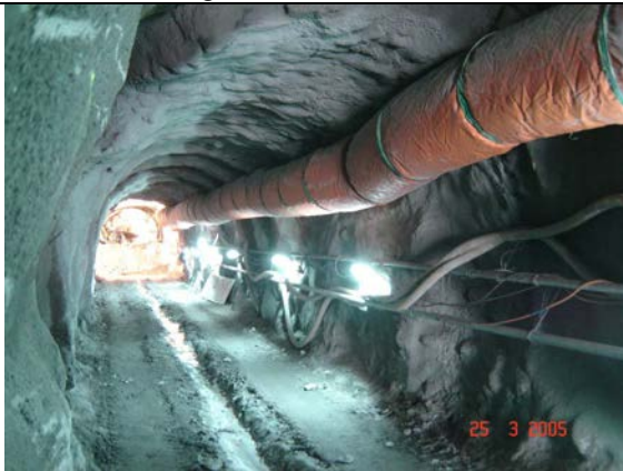
General View of Cable Tunnel Excavation
