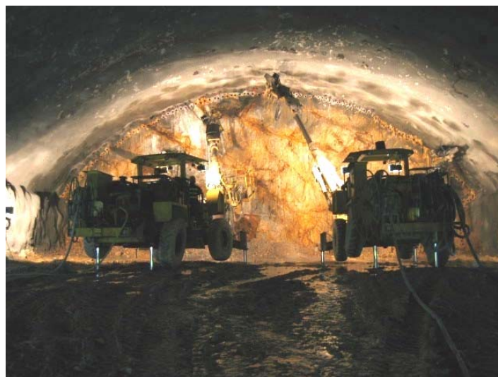
Plate 1: SWSR tunnel No. 2 top heading excavation
