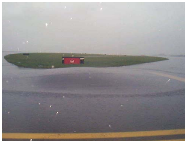
Figure 2: Heaving of pavement at the taxiway shoulder
