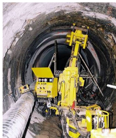
Drilling rig providing torque and support
