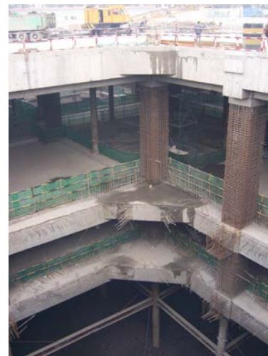
Figure 20: A view into an access opening showing the underground structure
