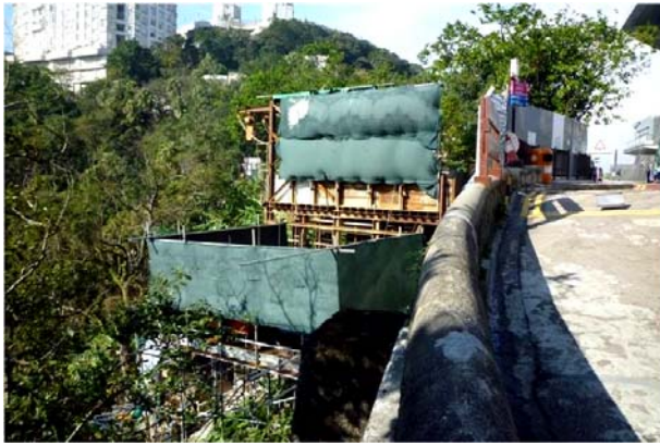
Plate 1: Temporary stockpiling platform
