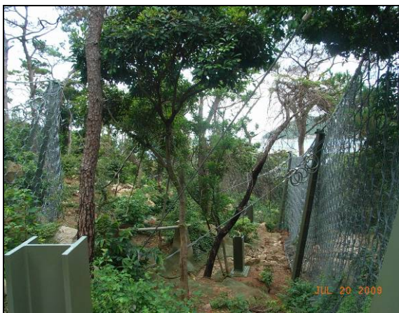
Plate 4: Flexible barriers and baffles erected at NC6
