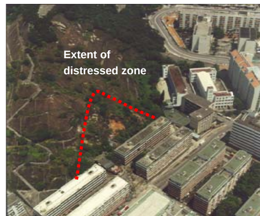
Figure 18: Landslide at Shek Kip Mei in 1999
