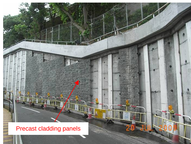
Plate 5: Coombe Road was reopened while installation of precast cladding panels was still in progress
