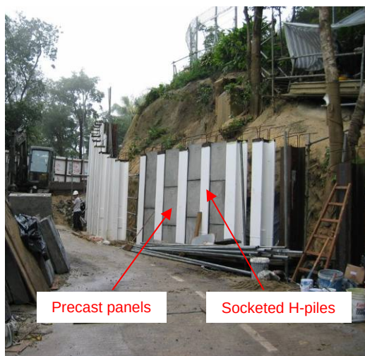
Plate 4: Construction of retaining wall
