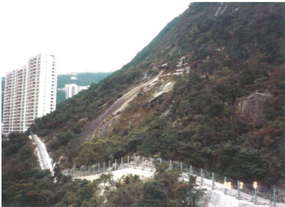
Figure 7: Boulder Fence at Mid-levels
