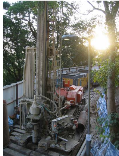
Plate 3: Congested works site during piling works
