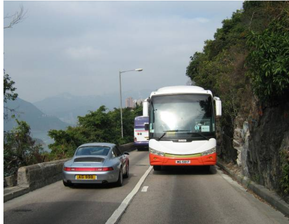
Plate 1: Typical narrow and busy road with cut slope, Repulse Bay Road, Hong Kong.
