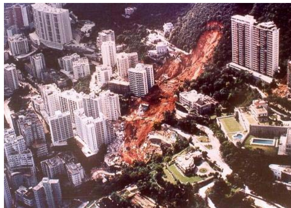
Figure 2: Landslide at Po Shan Road in 1972
