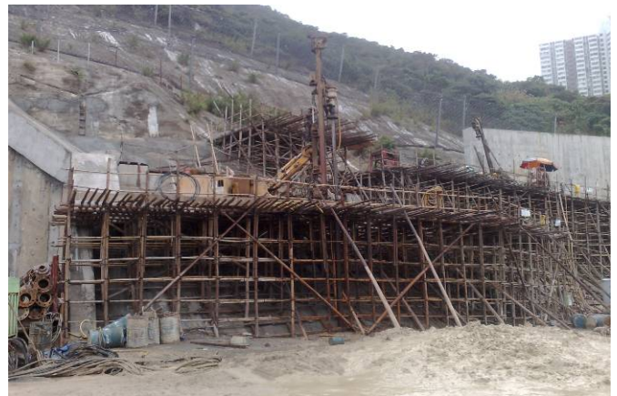
Plate 2: Bamboo scaffolding for mini-pile drilling rig
