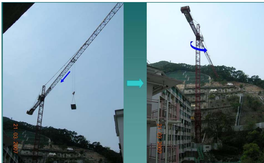
Figure 2: The operation procedure of tower crane presented in the Residents' Forum
