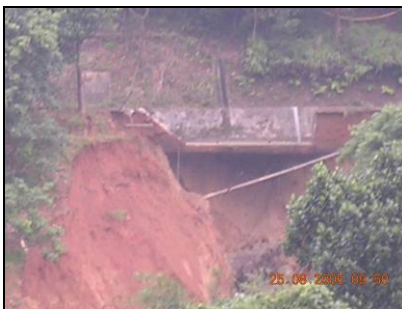
Plate 1: General view of slope failure
