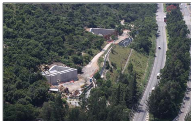
Figure 13: Existing condition during construction
