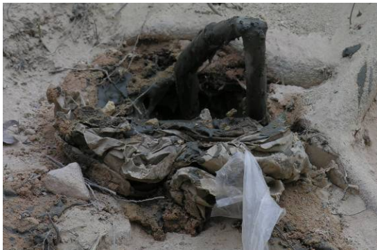
Plate 10: Top of drillhole plugged with cement package bags
