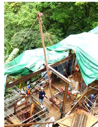
Plate 9: Lifting derrick
