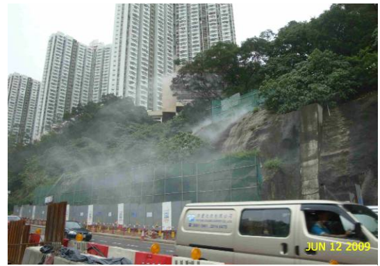
Plate 8: Dust coming out even with the use of tarpaulin sheet and water spraying
