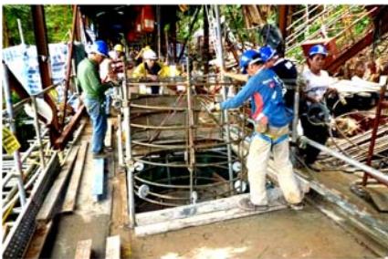
Plate 10: Reinforcement cage
