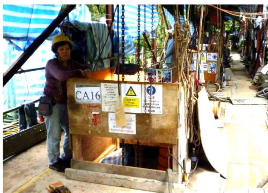
Plate 3: Provision of barriers and toeboards at caisson opening
