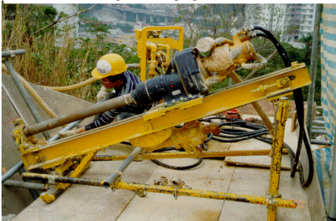
Plate 3 – Typical soil nail drilling rig with 1.5 m long leader
