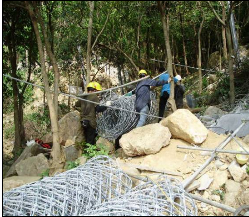
Plates 2 & 3: Manual handling of the wire mesh and steel baffle of flexible barrier at NC7a
