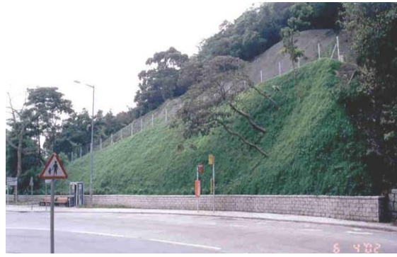
Plate 6: Slope with existing shotcrete surface before and after slope works including application of continuous fibre reinforced soil, Peak Road, Hong Kong
