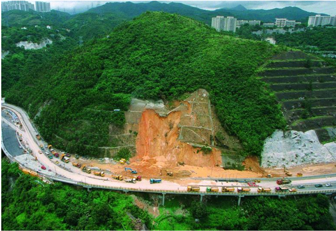
Plate 4: The Ching Cheung Road landslide in August 1997
