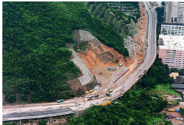
Figure 12: The 1997 Ching Cheung Road landslide
