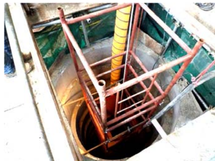
Plate 8: Climbing mast inside caisson
