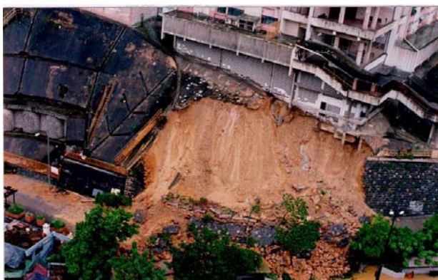
Figure 16: Kwun Lung Lau Landslide in 1994
