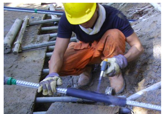
Plate 16: Use of hand-held blower to apply the heat-shrinkable mastic material onto the soil nail steel bar
