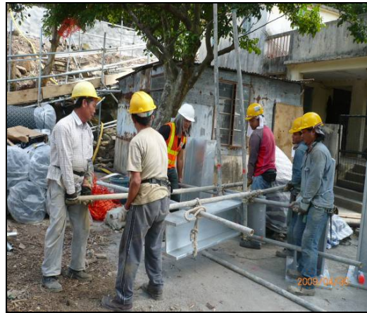
Plates 2 & 3: Manual handling of the wire mesh and steel baffle of flexible barrier at NC7a
