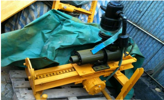
Plate 5: Special soil nail drilling rig with leader less than 1 m long
