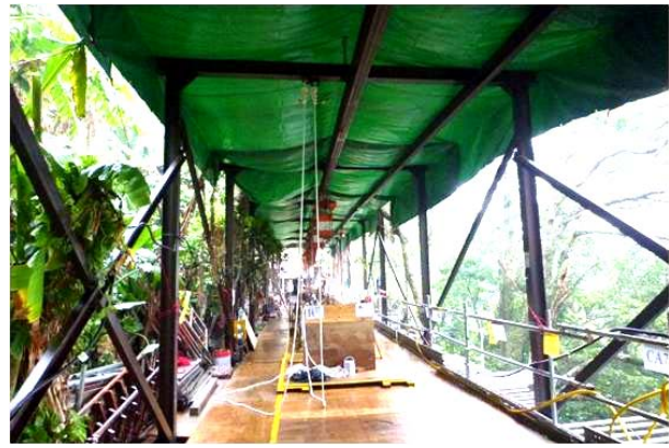
Plate 2: Temporary working platform and steel gantry
