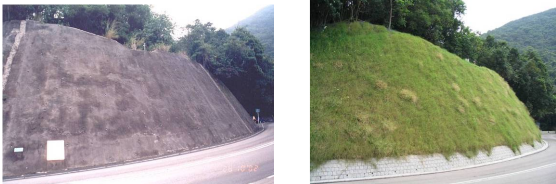
Plate 5: Slope with existing shotcrete surface before and after slope works, Stubbs Road, Hong Kong
