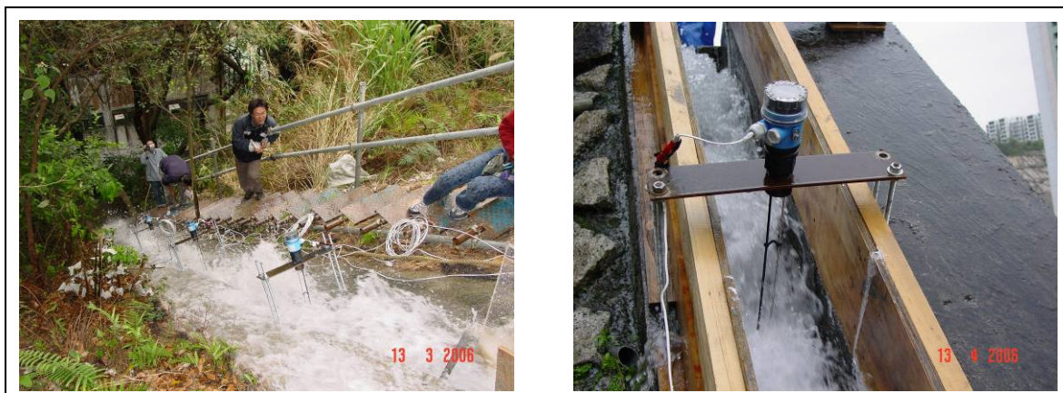
Figure 1: Field test of stepped drainage channel
