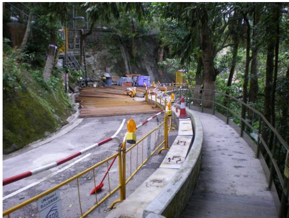
Plate 2: Temporary pedestrian walkway
