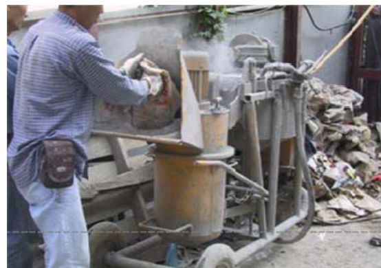
Plate 13: Smaller grouting equipment used for LPM site
