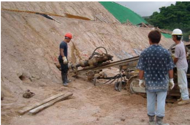
Plate 1: Use of mini-pile drilling rig for soil nail construction
