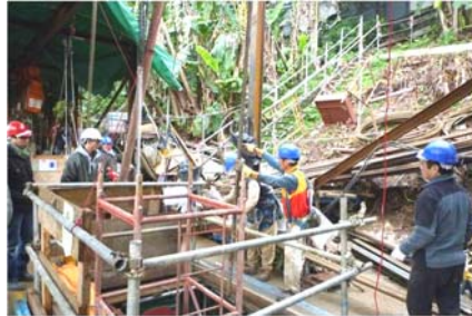
Plate 11: Lowering of 40mm dia. steel bar by lifting derrick
