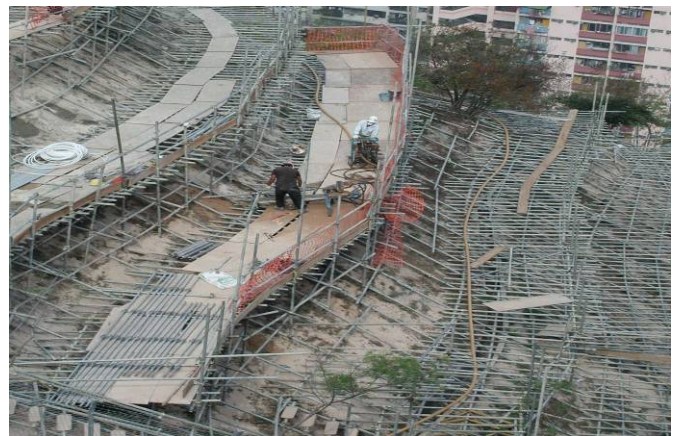
Plate 4: Steel tubular scaffolding for soil nail construction
