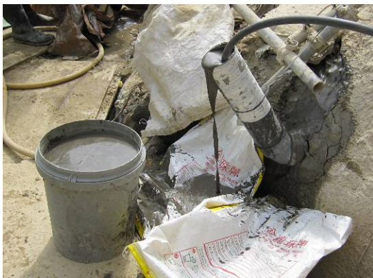
Plate 12: Use of “L-shaped” upstand pipe for maintaining grout level
