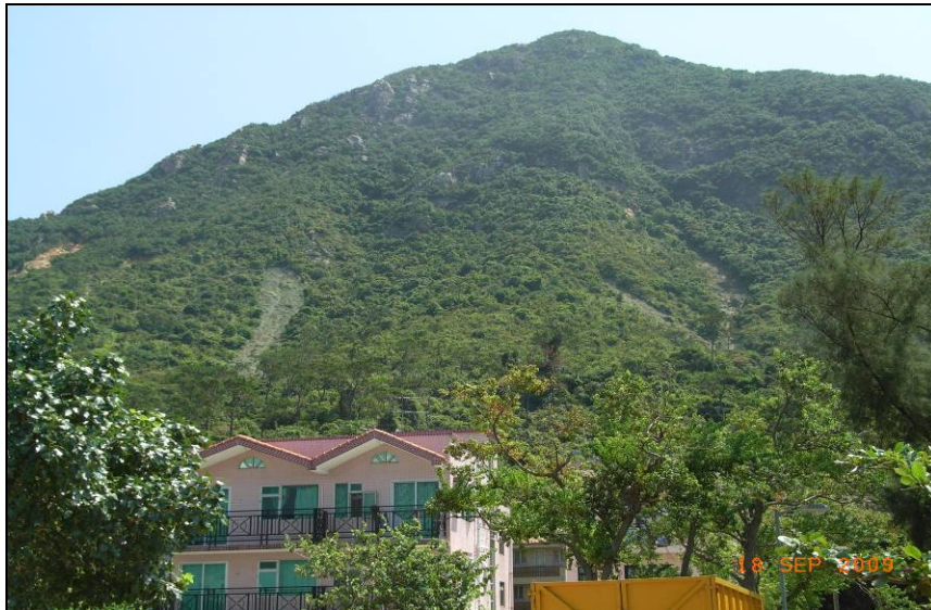
Plate 10: Completed landscaping works on slip scars of NC6 and NC7
