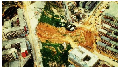
Plate 2: The June 1972 Sau Mau Ping landslide (71 fatalities)
