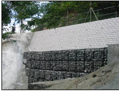
Plate 3: As-constructed remedial works
