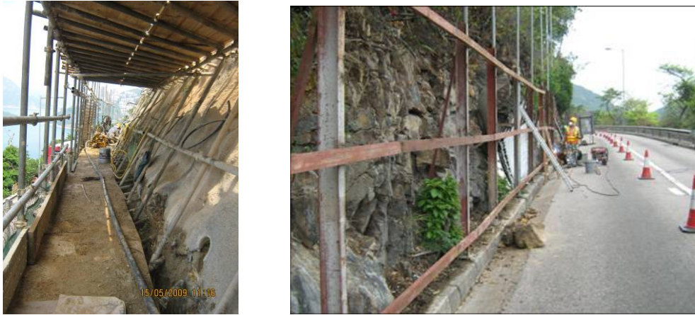
Plate 4: Temporary working platform, 1.1m width, Repulse Bay Road, Hong Kong
