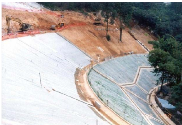
Figure 4: Recompaction of Loose Fill Slope
