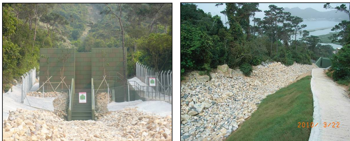
Plates 6 & 7: Completed RC check dam and re-profiled stream course at NC7
