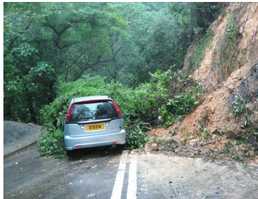
Plate 2: Landslide in weathered volcanic rock, Repulse Bay Road, Hong Kong, June 2008
