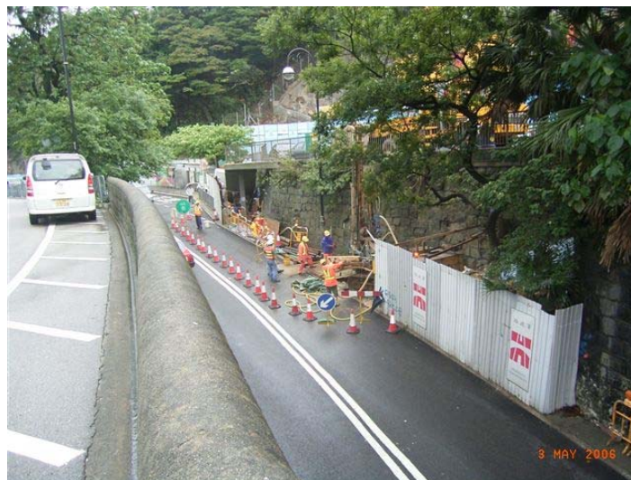
Plate 3: TTA for piling works at 11SW-C/R62 in Peak Road.
