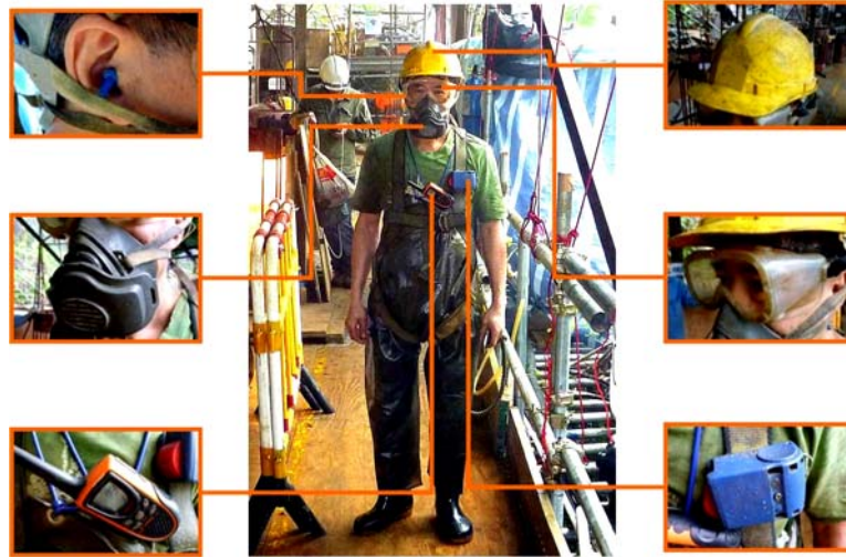
Plate 13: Personal protective measures for caisson workers
