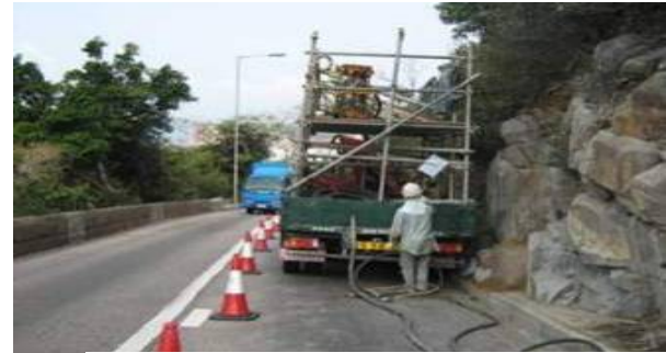
Plate 6: Drill rig on Lorry
