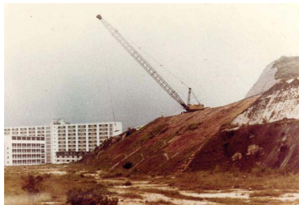
Figure 5: Dynamic Compaction of Loose Fill Slope (Lam 1980)
