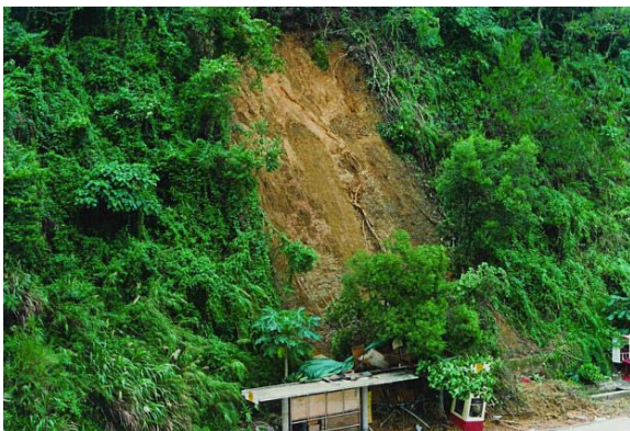
Figure 15: Landslide at Cheung Shan Estate Bus Terminus in 1993
