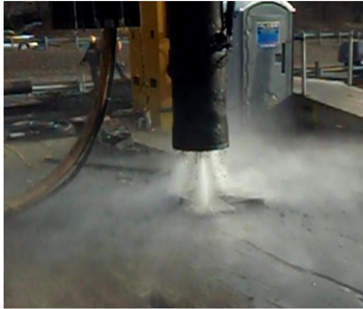
Figure 2: Water jet created by high pressure at outlet holes of drillbit
