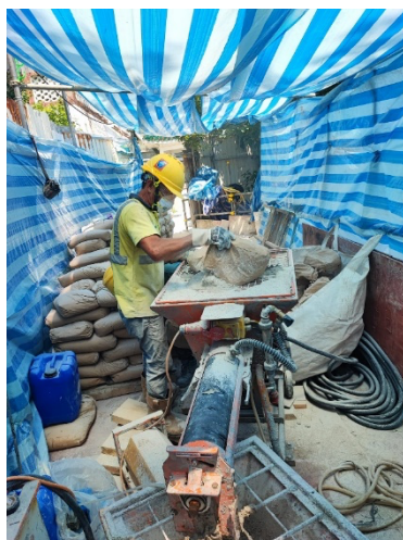
(a) Production of SCM using screw mixer on site
