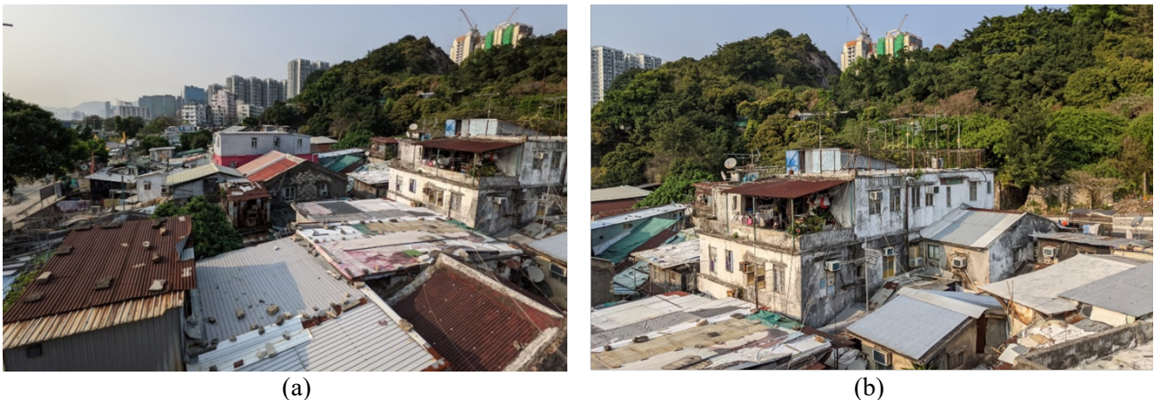
Figure 8: (a) Corrugated rooftop unsuitable for installation of GNSS rover station in CKL Village and (b) Rooftop occupied by antennas & prior consent from resident required for installing GNSS rover station
