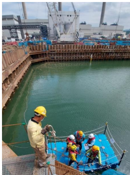
Plate 4: Confirmation of the Founding Level
