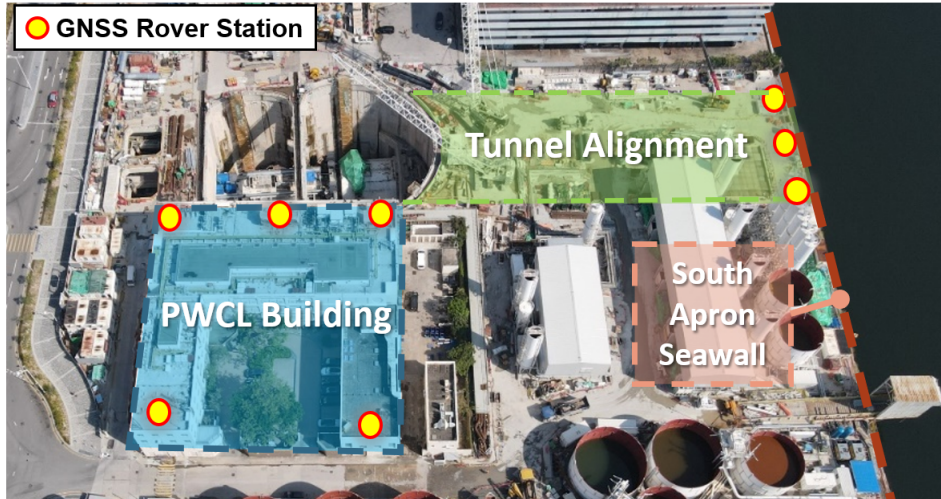
Figure 2: Phase 1 GNSS monitoring: at rooftop of PWCL Building (left) and along South Apron seawall (top right)
