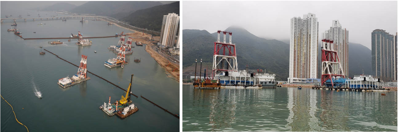
Figure 10: Marine DCM barges on work close to residential area
