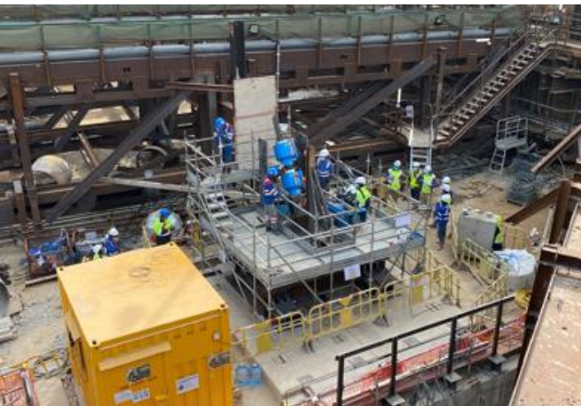
Figure 16: Ground Anchor Suitability Test Set Up
