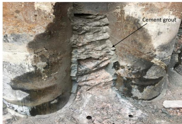
Figure 14: Grout observed in the rock socket during rock excavation
