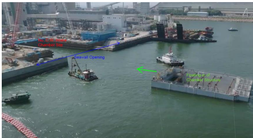
Plate 3: The EL with seawall opening for receiving the floating caisson
