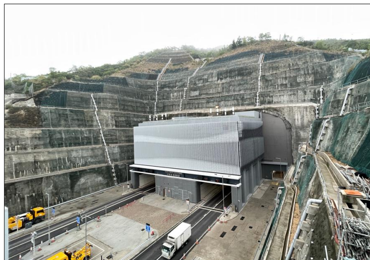
Figure 14: The completion of Semi-Cavern and EVB works
