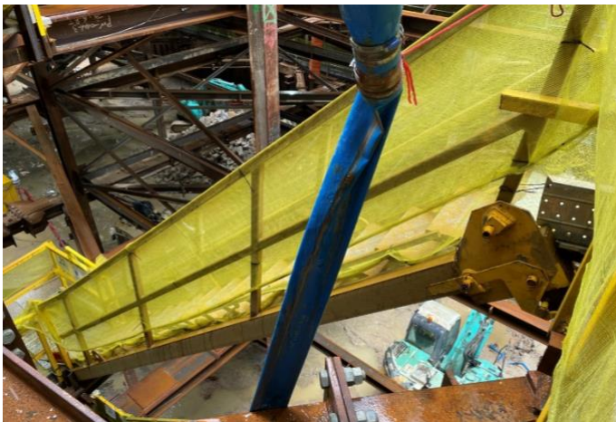
Figure 19 Actual Connection of the Modular Stair
