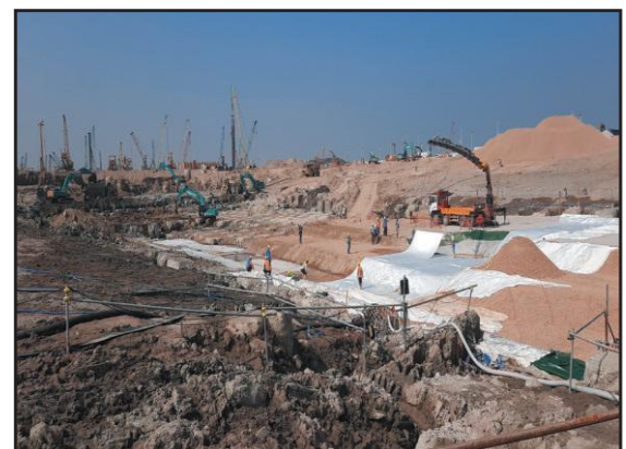
Reinforcement Geosynthetic Geotextile – 3 rd Runway Concourse, January 2022
