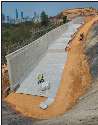
Geocomposite – Retaining Wall Drainage, Police Facilities Kong Nga Po, March 2021
