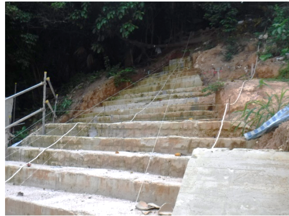
(b) Loose fill replaced by SCM
