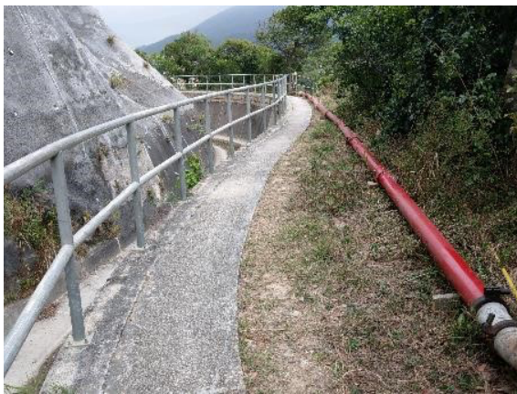
(c) Use of pipelines for transportation of SCM within the site
