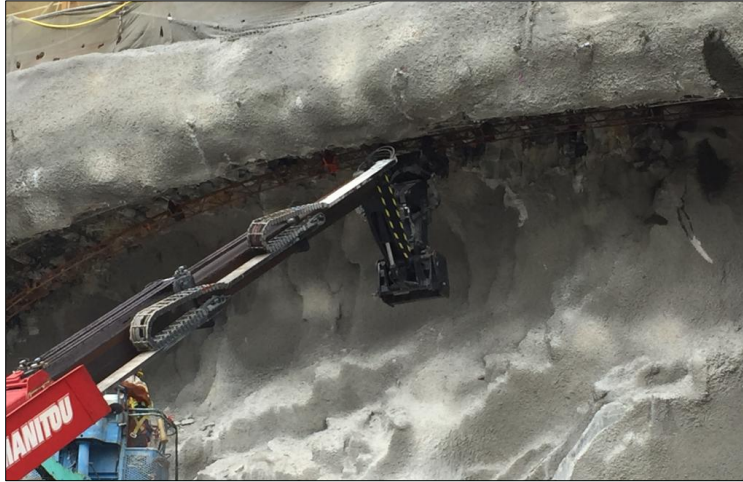
Figure 11: Installation of Lattice Girder Segment
