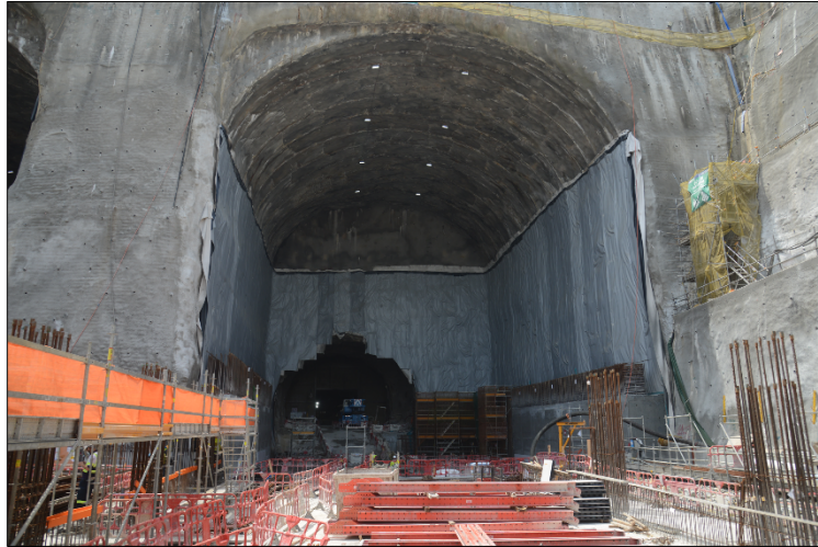
Figure 13: Waterproofing and Reinforced Concrete Lining at Side Walls
