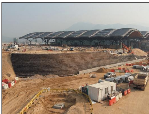
Geogrid - Reinforced Fill Slope HKZMB, October 2017
