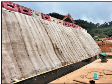
Concrete Canvas – Slope Work Kardoorie Farm, March 2020
