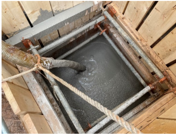
(a) Placement of SCM for fill replacement in a pit
