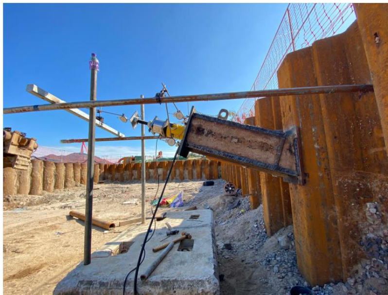
Plate 2: Set up of Pull out test on Site
