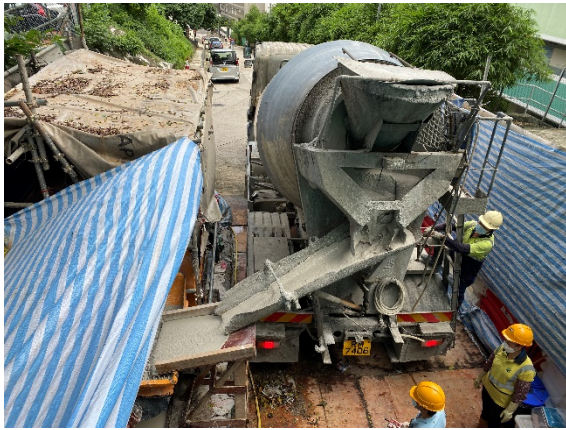
(a) Delivery of ready-mixed SCM by concrete truck
