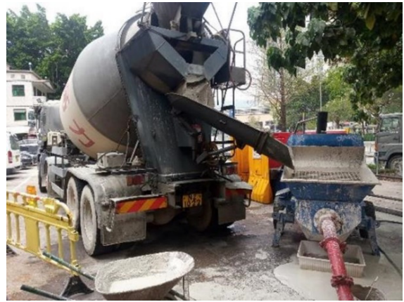
(b) Discharge of ready-mixed SCM to concrete pump
