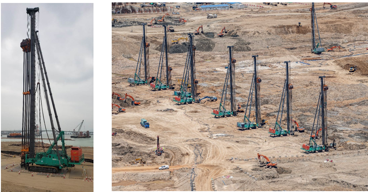
Figure 15: Land DCM machines and its working on land
