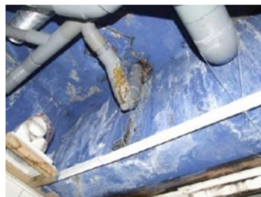
Figure 2. Microbial and bacterial growth in the ceiling.
