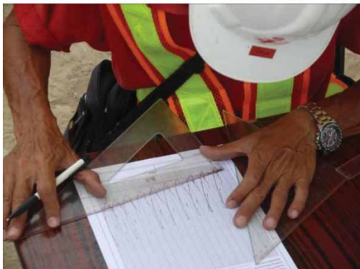
Figure 2. Final set graph by manual method: (a) drawing final set graph by a worker holding a pencil in close proximity to a driven H-pile and (b) interpreting the results.
