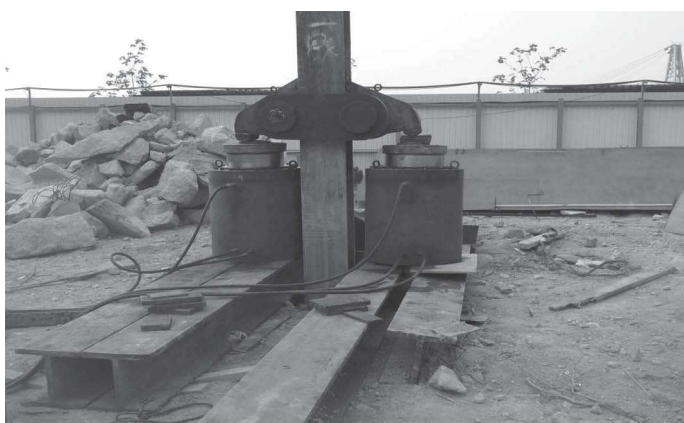
Figure 8 – Extraction of H-pile by Hydraulic Jack
