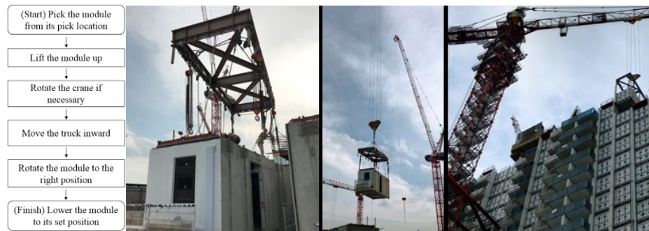
Figure 2. Module lifting process (Photo courtesy: Teambuild).
