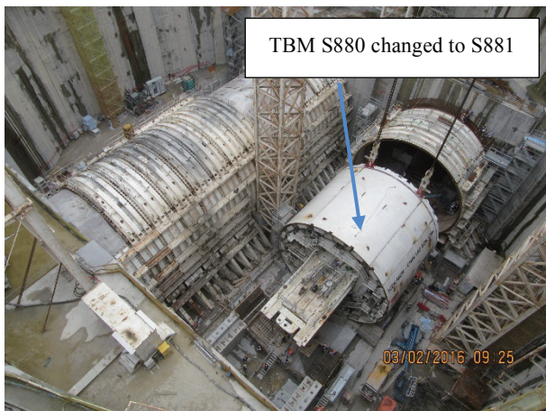
Figure 10. TBM (S880) changing diameter to TBM (S881).
