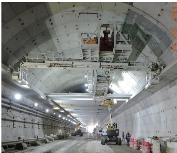
Figure 16. OHVD slab installation.
