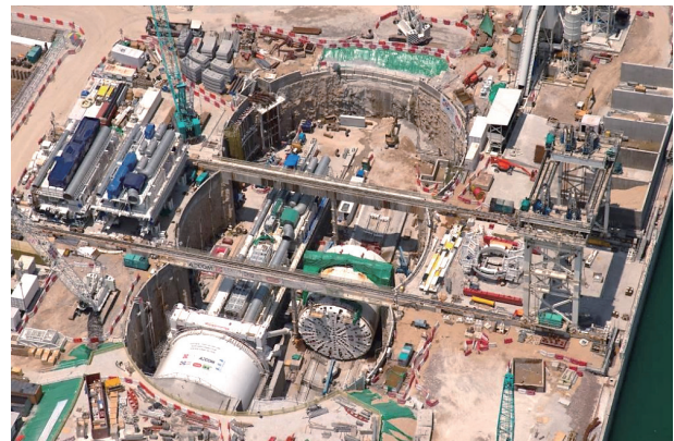
Figure 9. TBMs (S880) and (S882) assembly in the peanut-shaped LS.
