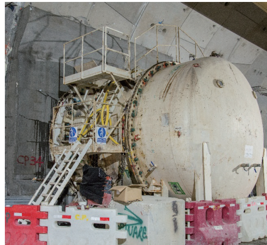
Figure 18. Receiving bell for MTBM break-out.
