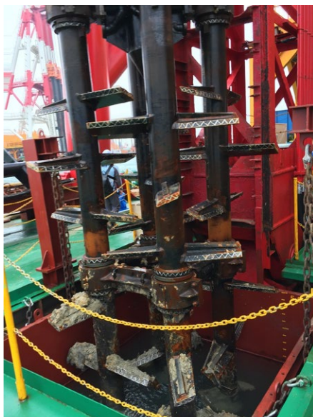
Figure 9. Augers of a drill rig on DCM barge.
