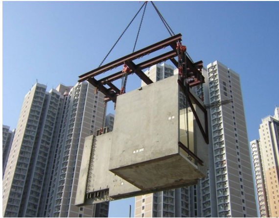
(a) Lifting a precast unit
