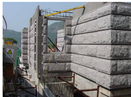
Figure 3.11 Decorative finishes on precast façade with granite cladding.
