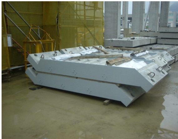
(a) Precast staircase
