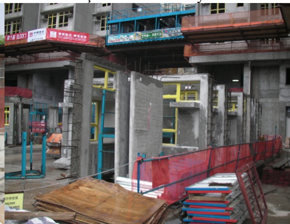
Figure 3.21 Proper storage to avoid excessive stresses and possible damage to precast units.
