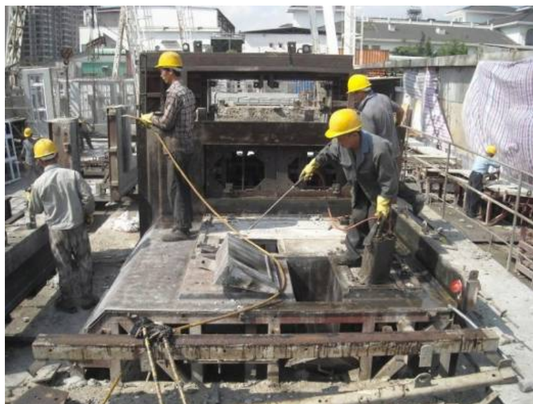
Figure 3.2 Applying mould release agent.
