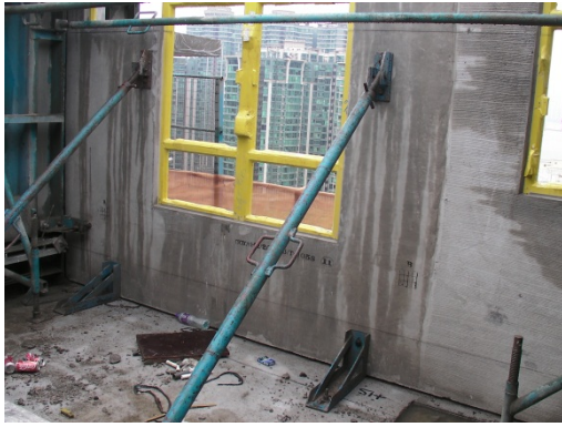
Figure 3.33 Verticality of precast façade adjusted to erection tolerances (right: levelling shim).
