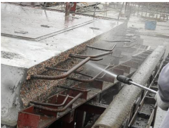
Figure 3.12 Water-washed finishes at the connection.
