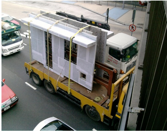
Figure 3.30 Ensure no undesirable stresses to the precast elements due to flexing of truck.
