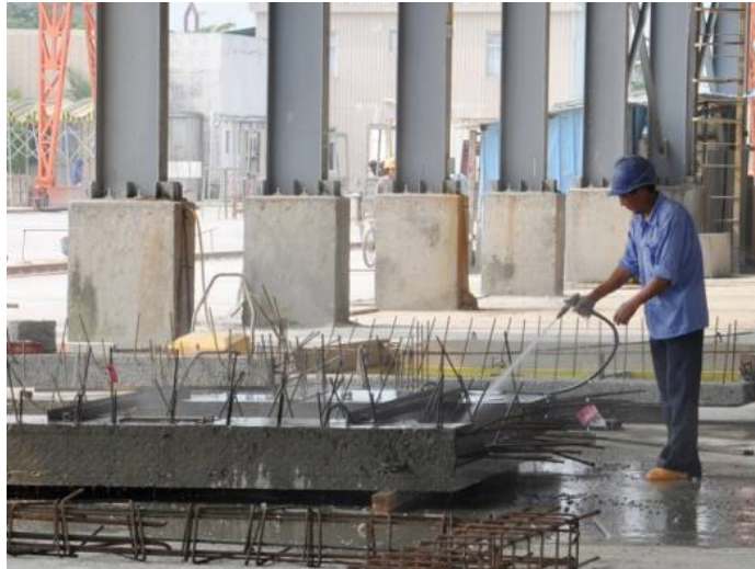
Figure 3.18 Application of water to precast unit for normal curing.
