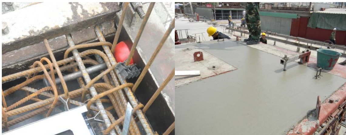
Figure 3.8 Examples of lifting inserts.
