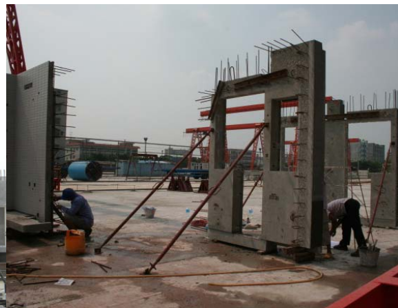
Figure 3.20 Temporary supports for façade in the factory.
