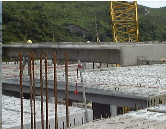
(b) Double-Tee panel slab
