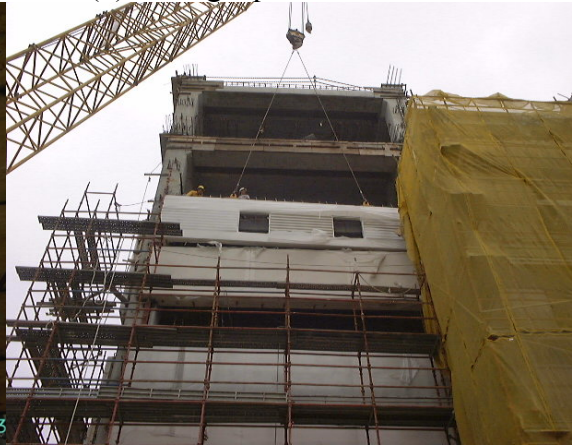
(c) Lifting a precast facade
