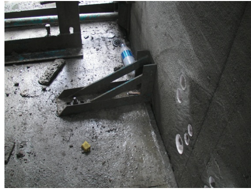
Figure 3.33 Verticality of precast façade adjusted to erection tolerances (right: levelling shim).
