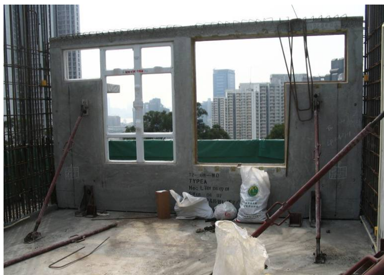
Figure 3.38 Method of erection for precast façade.
