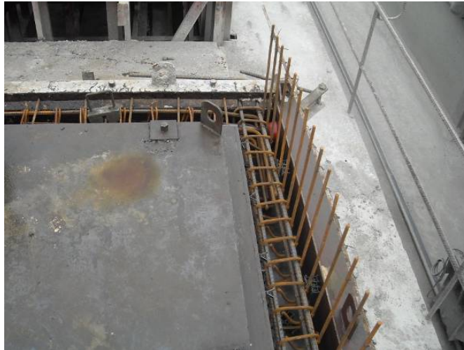
Figure 3.14 Checking of rebar, lap length, cover and lifting inserts before concreting.
