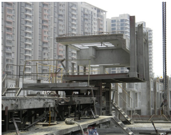
Figure 3.19 Rotatable steel rack for ease of lifting.
