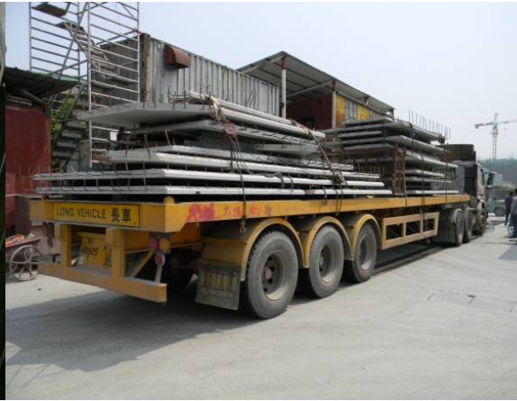
Figure 3.31 Pre-plan sequence of lifting to avoid multiple handling of precast elements.
