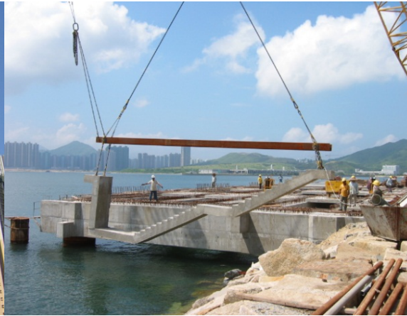
(b) Lifting a precast staircase
