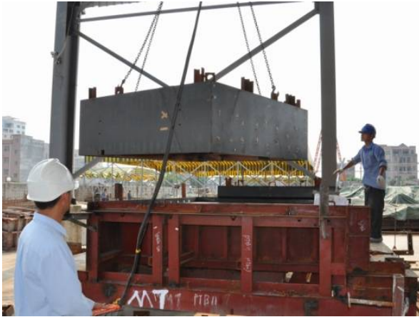
Figure 3.3 Steel mould with specified roughness and precision.
