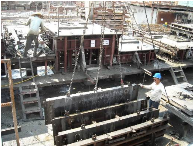
Figure 3.16 Detaching the mould from a precast element.
