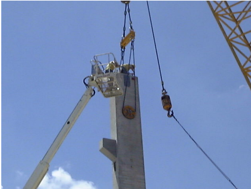
Figure 3.25 Example of lifting pin for a 30 ton precast column.
