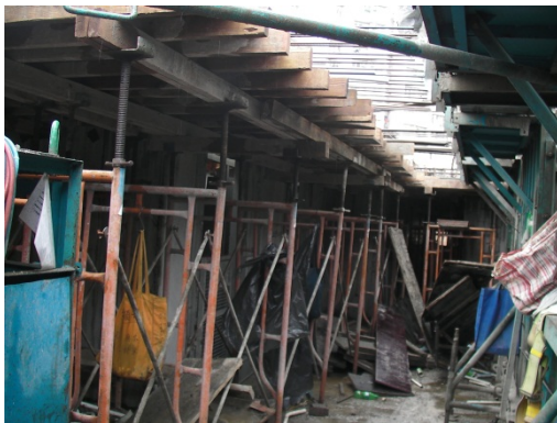
Figure 3.34 Proper popping and temporary support.
