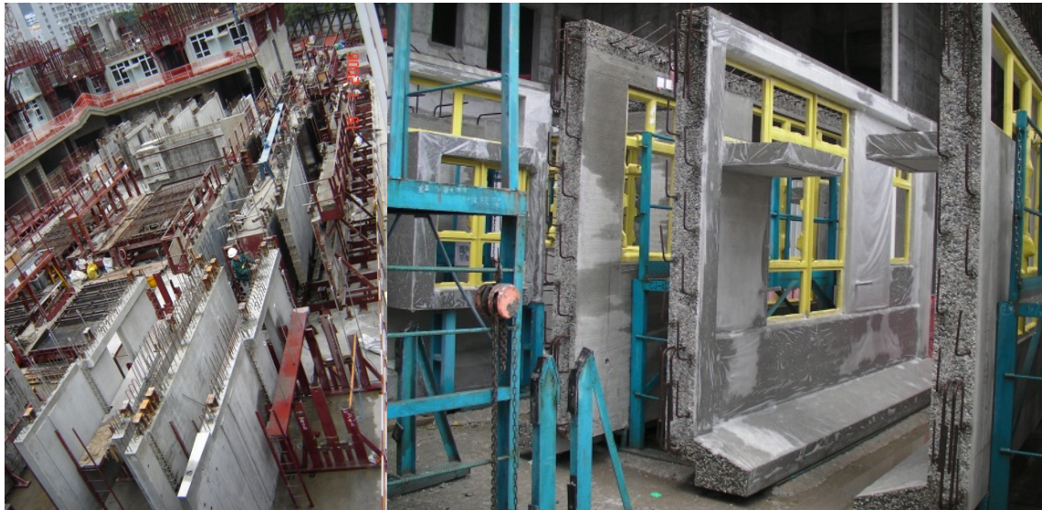
Figure 3.26 Precast units must be stored safely with adequate supports.
