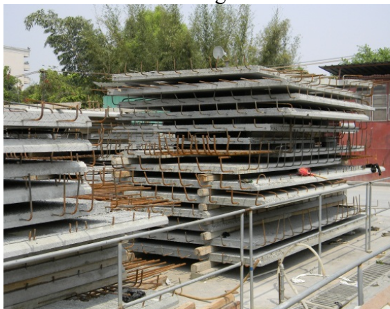
Figure 3.21 Proper storage to avoid excessive stresses and possible damage to precast units.
