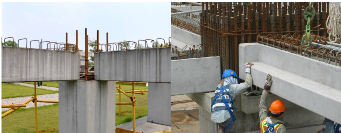
Figure 3.7 Cast-in connection on beams and columns.
