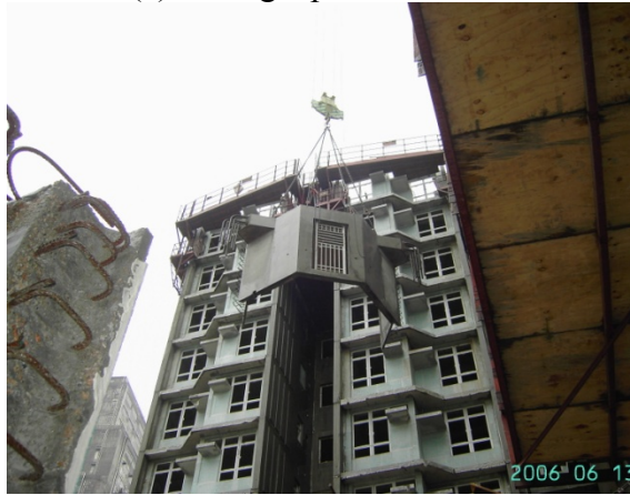
(c) Lifting a precast facade
