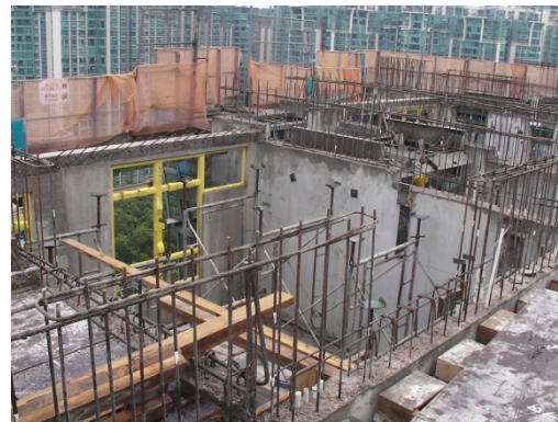
Figure 3.34 Proper popping and temporary support.
