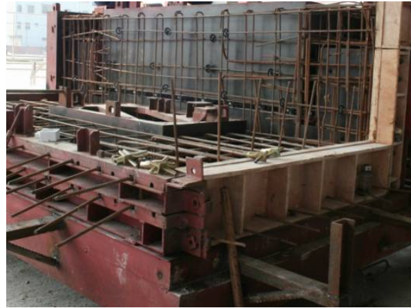
Figure 3.4 Combined use of steel mould and timber mould.
