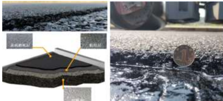
High performance asphalt pavement
