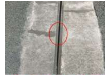
Rubber Cracking
