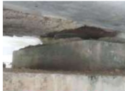
Rubber Cracking
