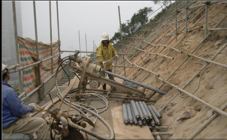
Use of soil nails to enhance the robustness of slope
