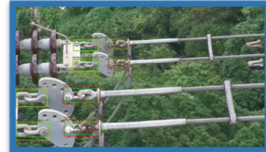
Pylon Tower / Radio Station Inspection
