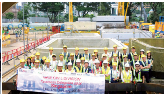
Singapore Delegation Site Visit to MRT Contract T221 Havelock Station (CV)
