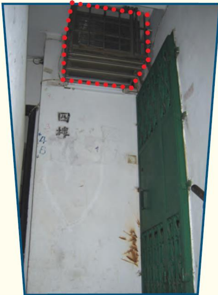
Opening formed in the staircase enclosure wall
