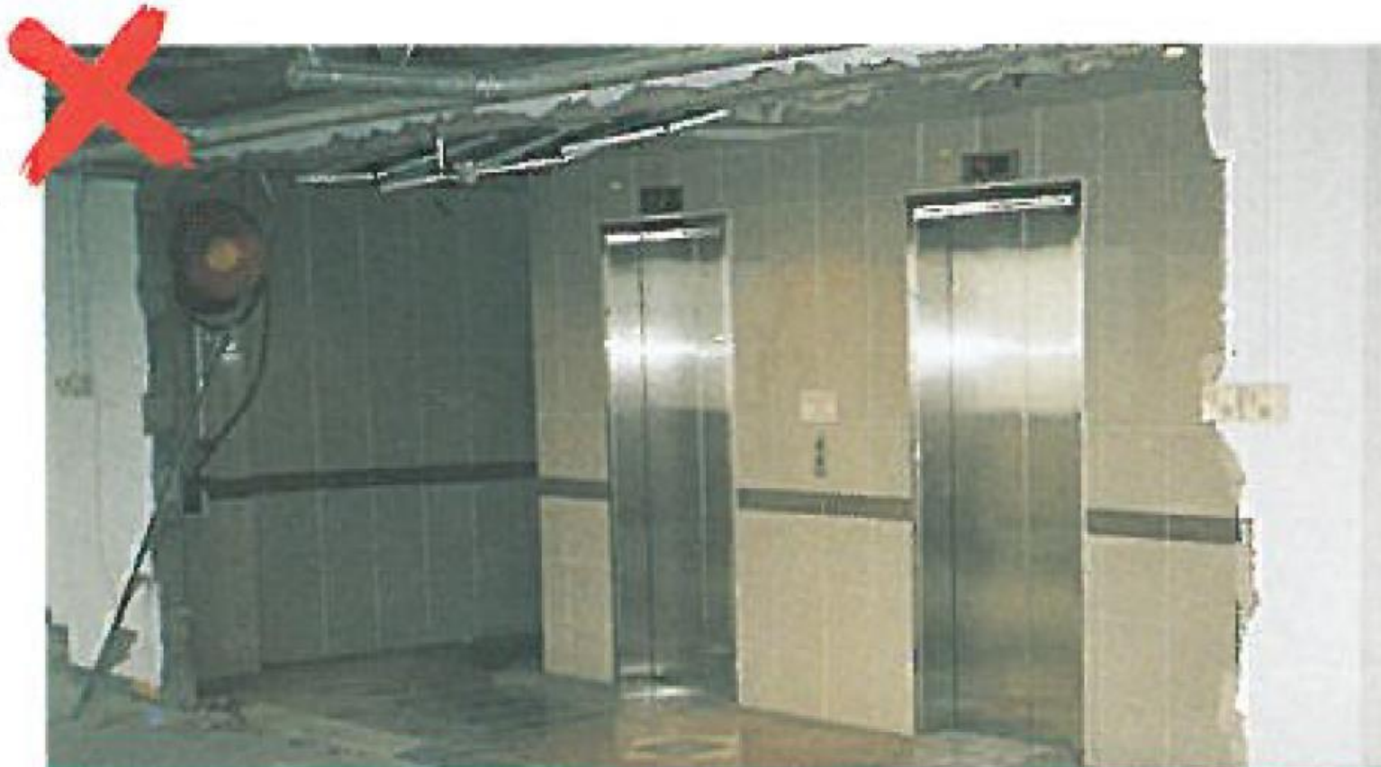
Removal of fireman's lift lobby
