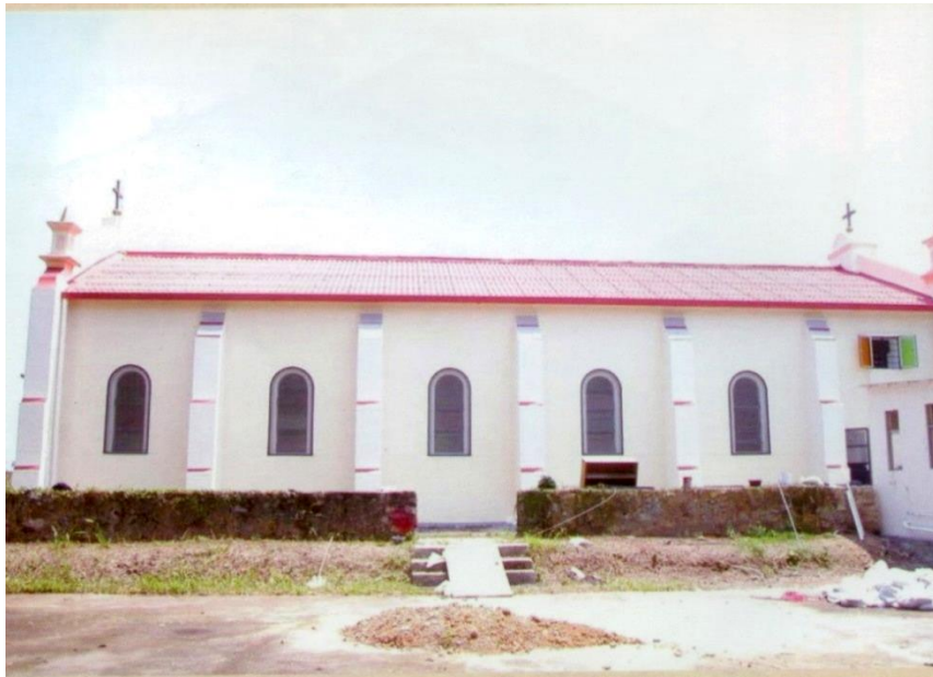
North-Western elevation of the Chapel after renovation
