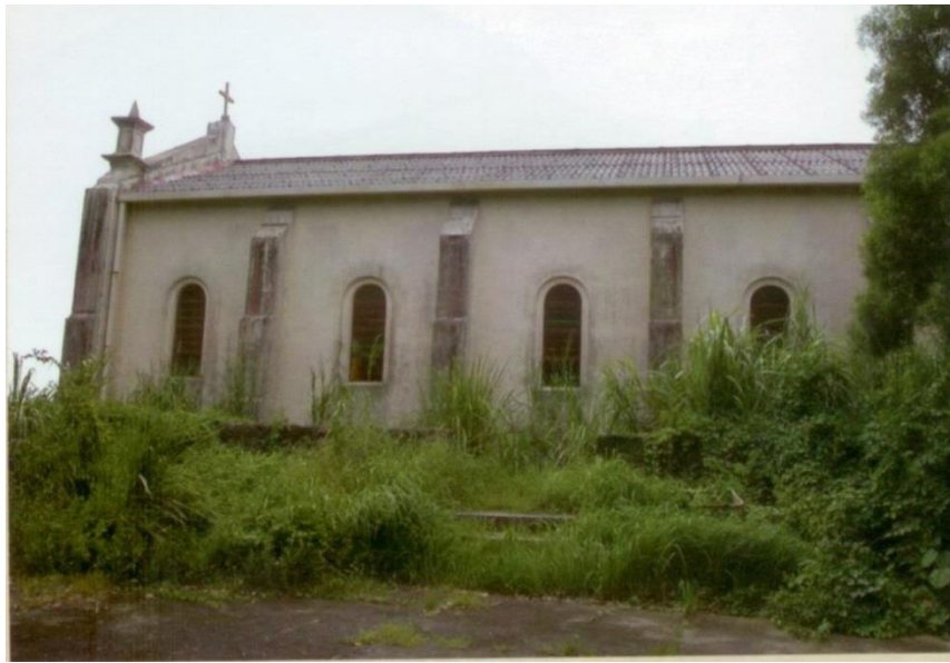
North-Western elevation of the Chapel before renovation
