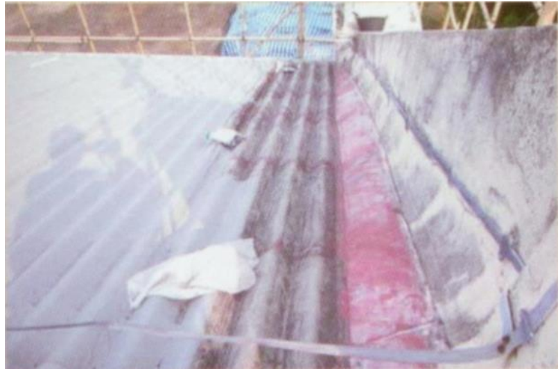
Waterproofing work to roof in progress
