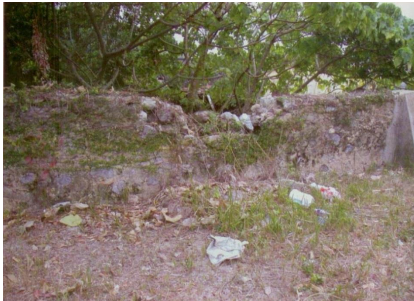
Parapet wall to the courtyard of the Chapel before repair
