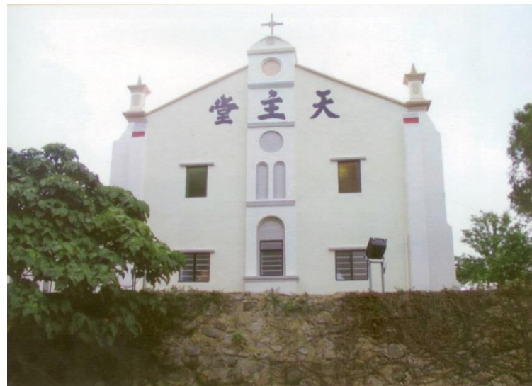
Rear elevation after renovation
