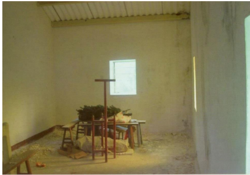
Priest's dormitory at mezzanine floor before renovation
