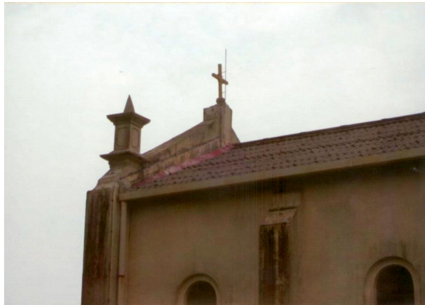
Roof before renovation
