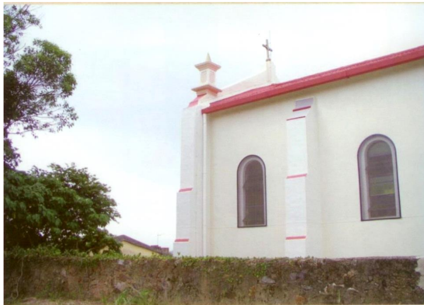
Roof after renovation
