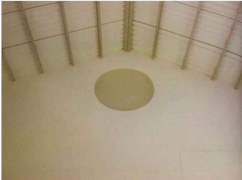
Soffit of the roof after renovation
