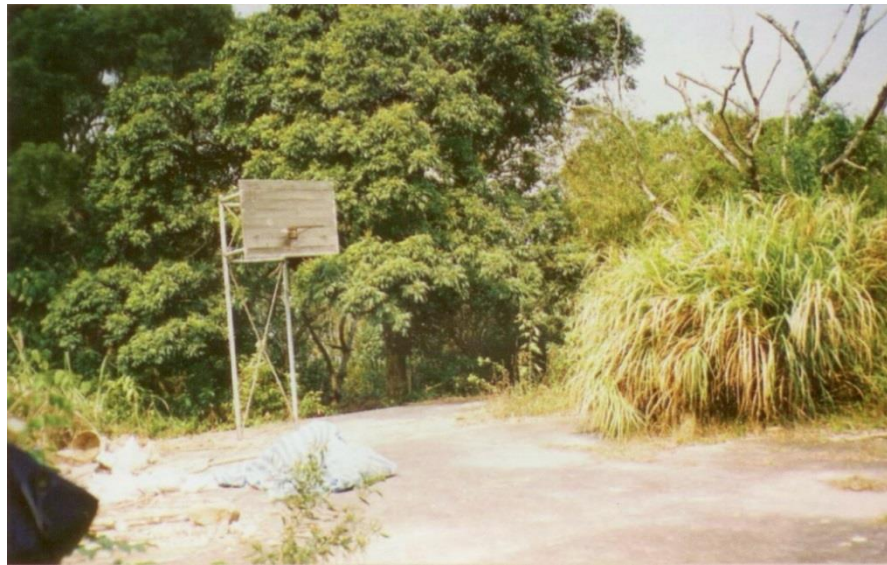
Basketball court before renovation
