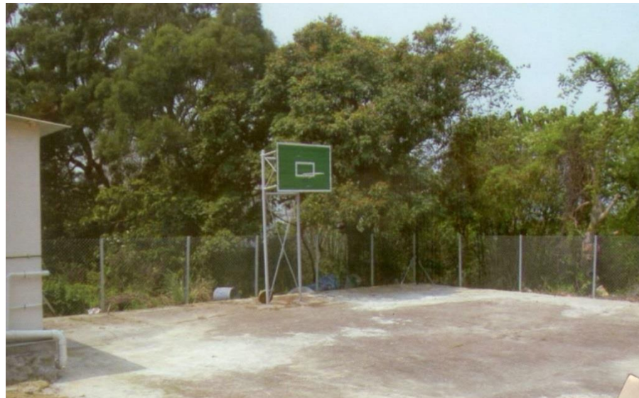
Basketball court after renovation
