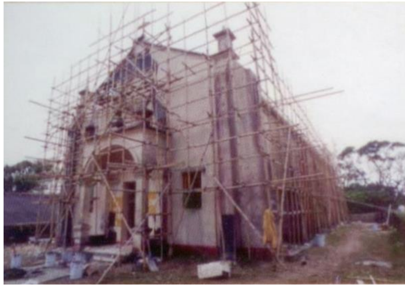
Bamboo scaffolding erected prior to the repair and renovation works
