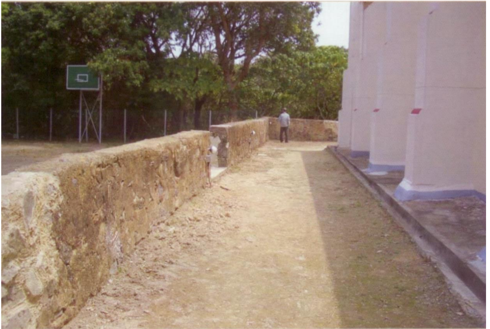
The stone parapet at the courtyard of the Chapel
