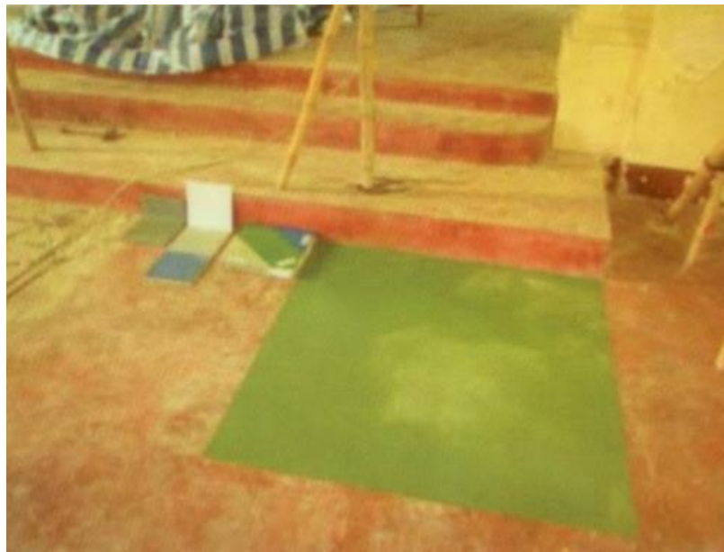
Repair of floor finishings, in the stage of colour scheming
