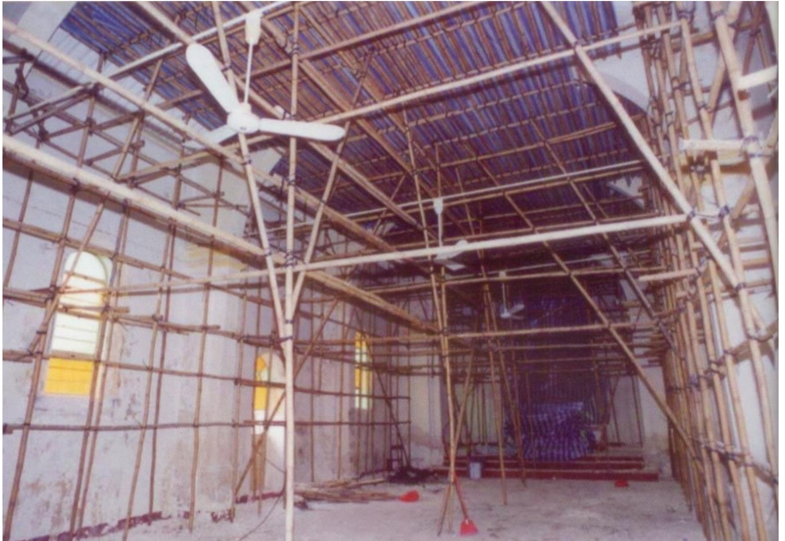
Bamboo scaffolding erected in the interior of the Chapel
