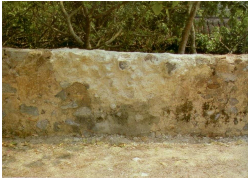
Parapet wall after repair
