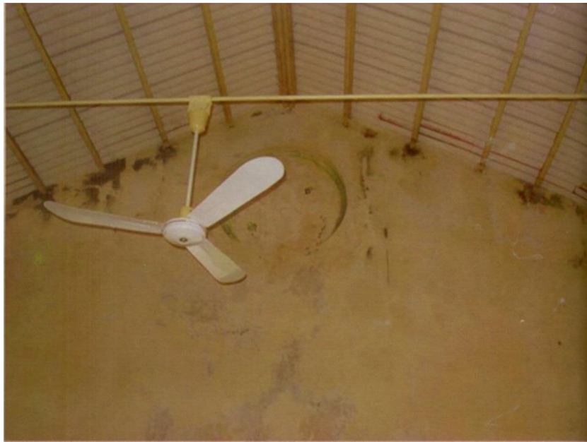
Soffit of the roof before renovation
