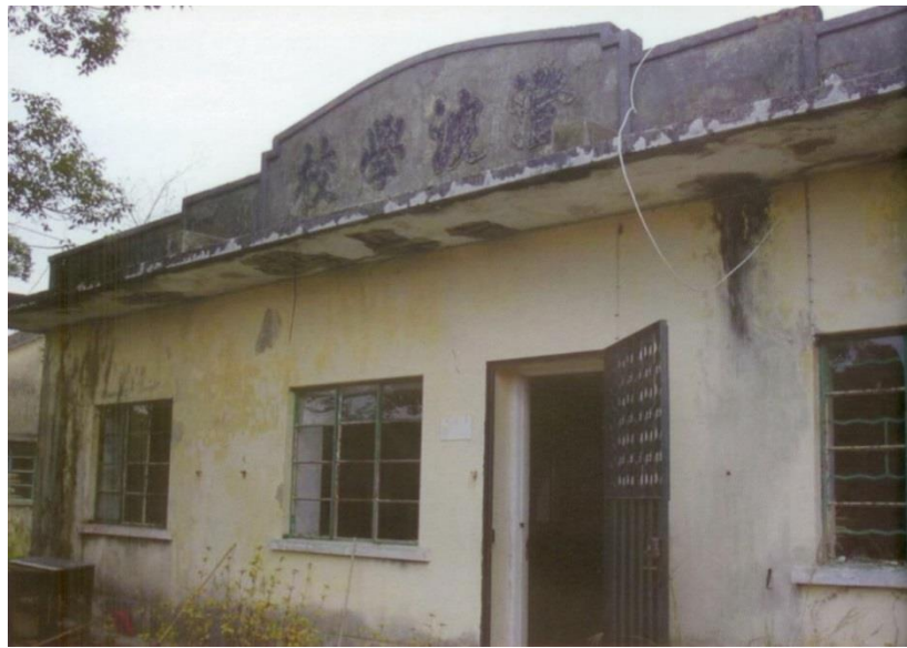
The abandoned Ching Po School before renovation
