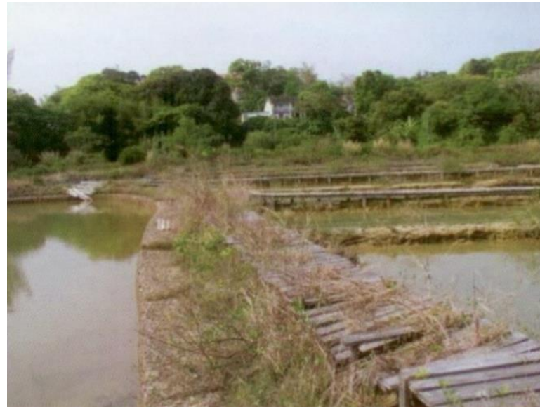
Timber planks on the access path to various locations of the salt fields
