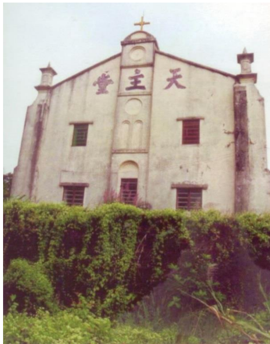
Rear elevation before renovation
