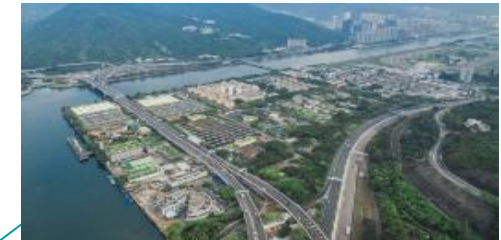
Relocation of Sha Tin Sewage Treatment Works to Caverns
