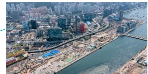
Trunk Road T2 and Cha Kwo Ling Tunnel
