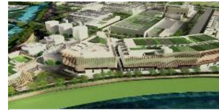
Shek Wu Hui Effluent Polishing Plant
