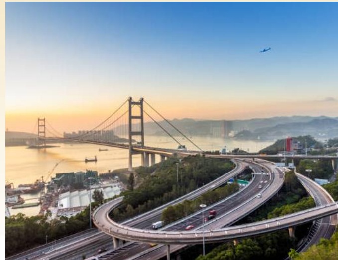
Tsing Ma Bridge
