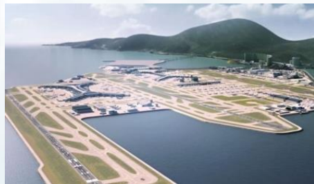
Three Runway System Project
