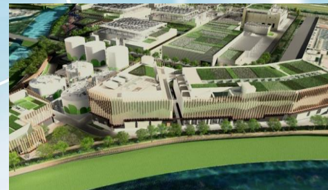
Shek Wu Hui Effluent Polishing Plant
