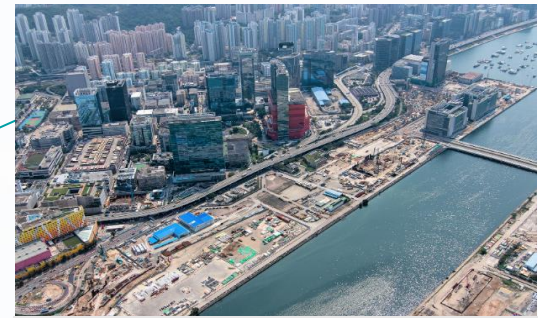
Trunk Road T2 and Cha Kwo Ling Tunnel
