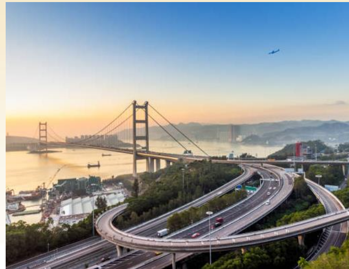
Tsing Ma Bridge
