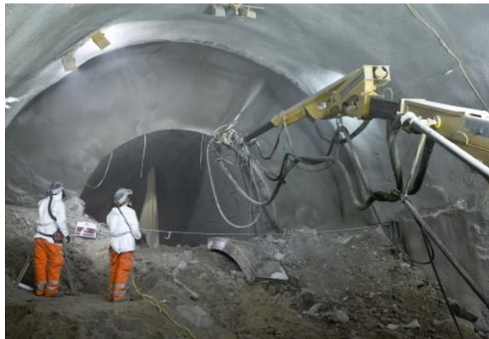
Vibration Resisting Concrete Lining in Cavern Construction
