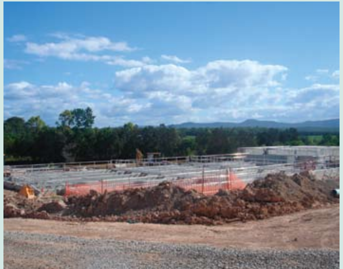
Fig C4.11 General View of the construction site of the wastewater treatment plant
