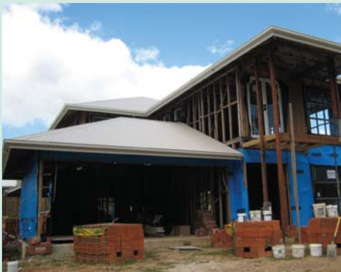
Fig C4.7 A new house in Coommera Estate under construction
