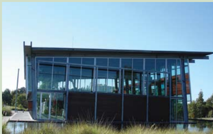
Fig C1.10 Water Treatment Plant in Sydney Olympic Park
