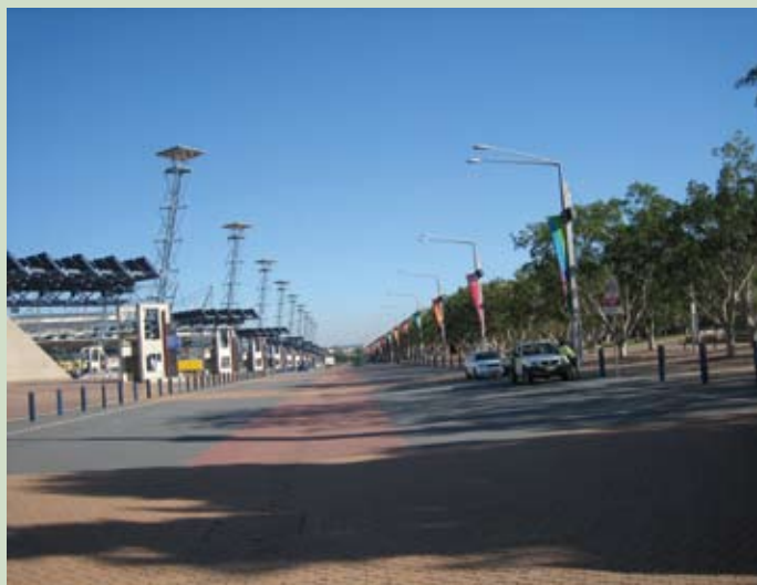
Fig C1.11 Photovoltaic towers lining Olympic Boulevard
