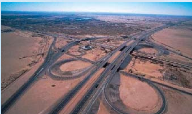
Figures 3.3.5 Construction of road interchanges [4]
