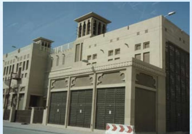
Figure 3.1.15 Harmonized power substation design (U) with luxury houses (D) on Palm Jumeirah
