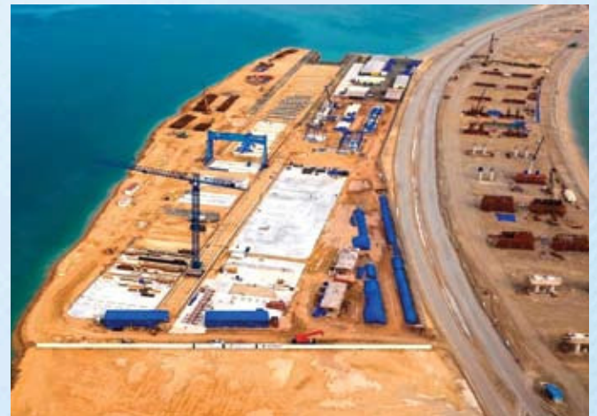
Figure 3.4.20 Precasting yard for Water Home platforms and entrance bridge beams [19]
