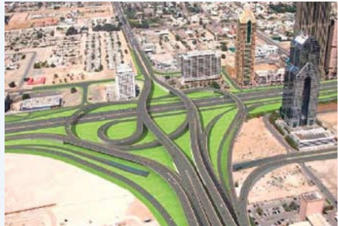
Figures 3.3.6 Construction of road interchanges [4]
