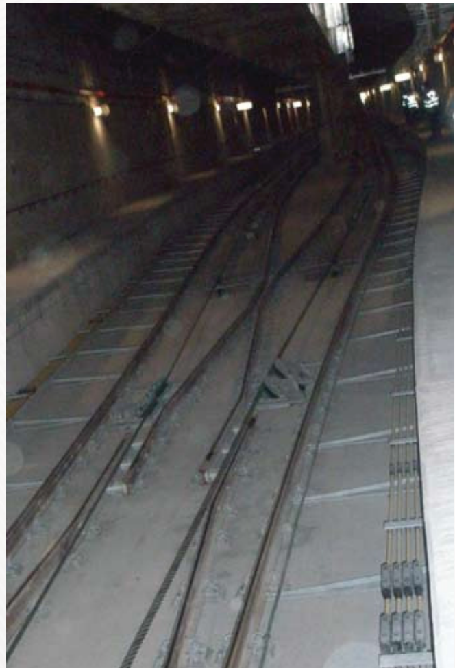
Figure 6.6 Funicular tunnel with passing loop
