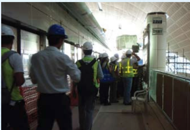
Figure 3.1.14 Project engineers explaining building services design at station platform
