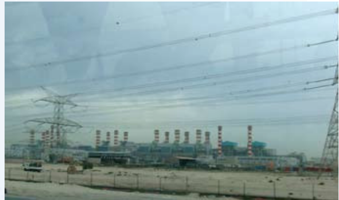
Figure 3.3.23 DEWA's power and desalination plant
