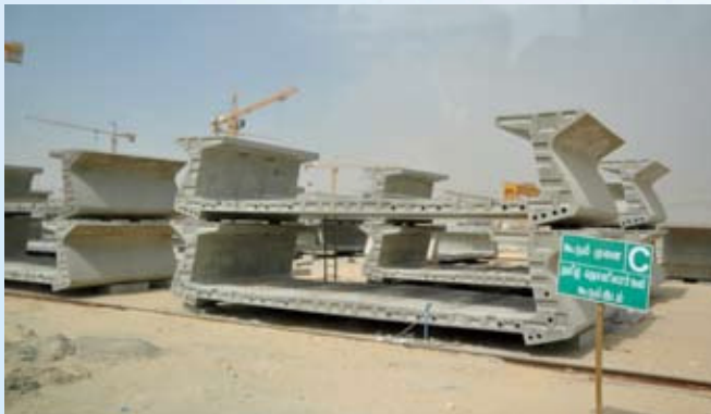
Figure 3.1.10 Pre-casted rail segments
