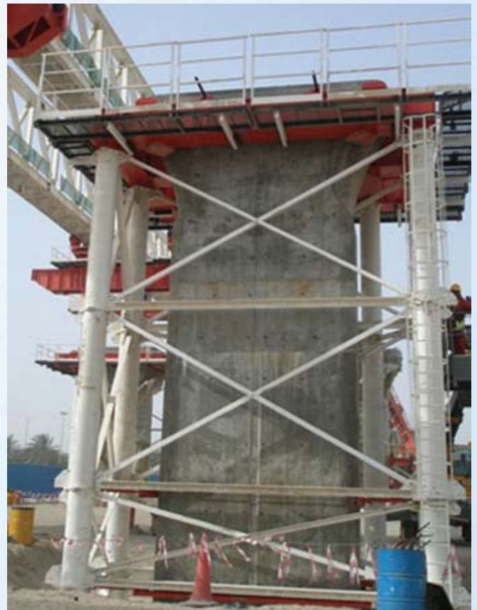
Figure 3.3.21 Temporary steel tower for segments
