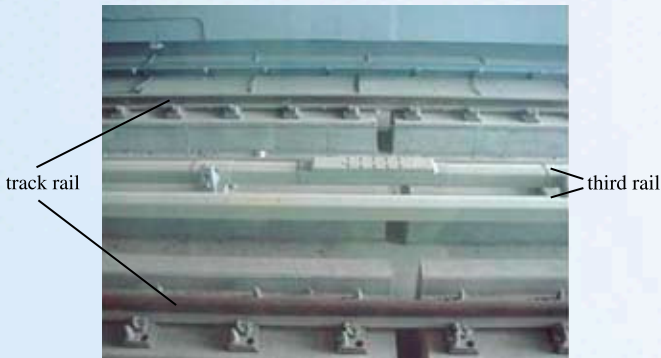
Figure 3.3.16 Third rail in Dubai Metro
