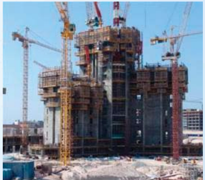
Figure 3.4.10 Construction of Burj Dubai showing the climbing formwork [10]
