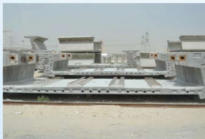
Figure 3.3.12 Precast segments at Dubai Metro precasting yard
