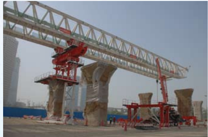
Figure 3.1.12 Launching gantry at RTA major road project construction site
